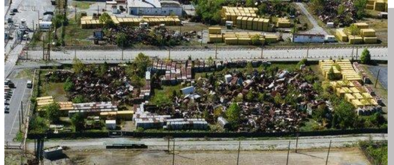
This old scrap yard at Y-12 will be one of the first cleanup projects to be done with stimulus money in Oak Ridge.
