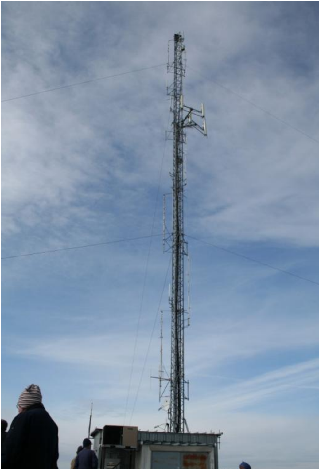
Figure A.17. Crown Castle Building and Tower (Locale 5). Photo taken at 250 degrees on 3/19/09 by Doug McFarland.
