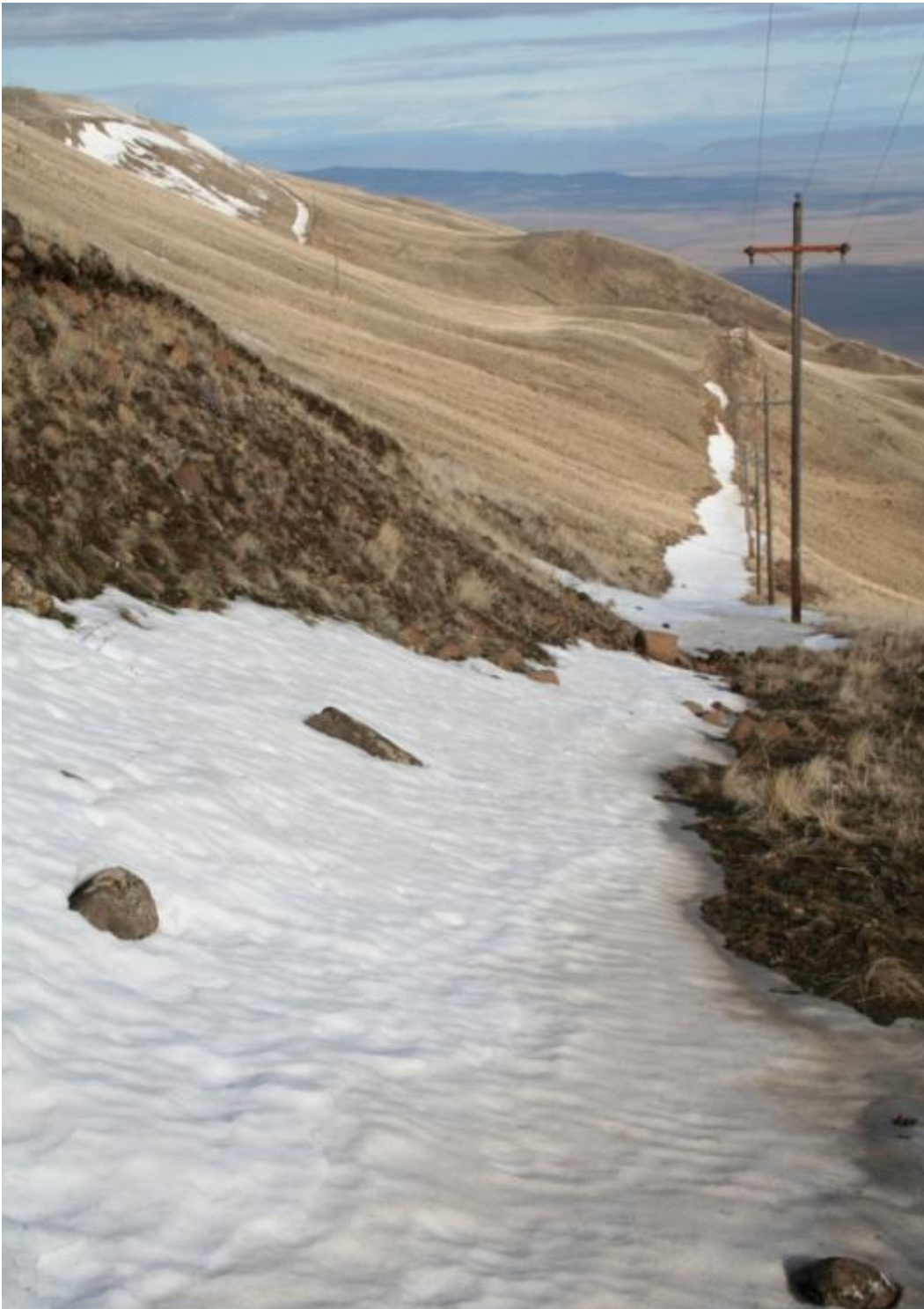
Figure A.42. Benton PUD Electrical Line (Locale 9A). Photo taken at 330 degrees on 3/20/09 by Doug McFarland.
