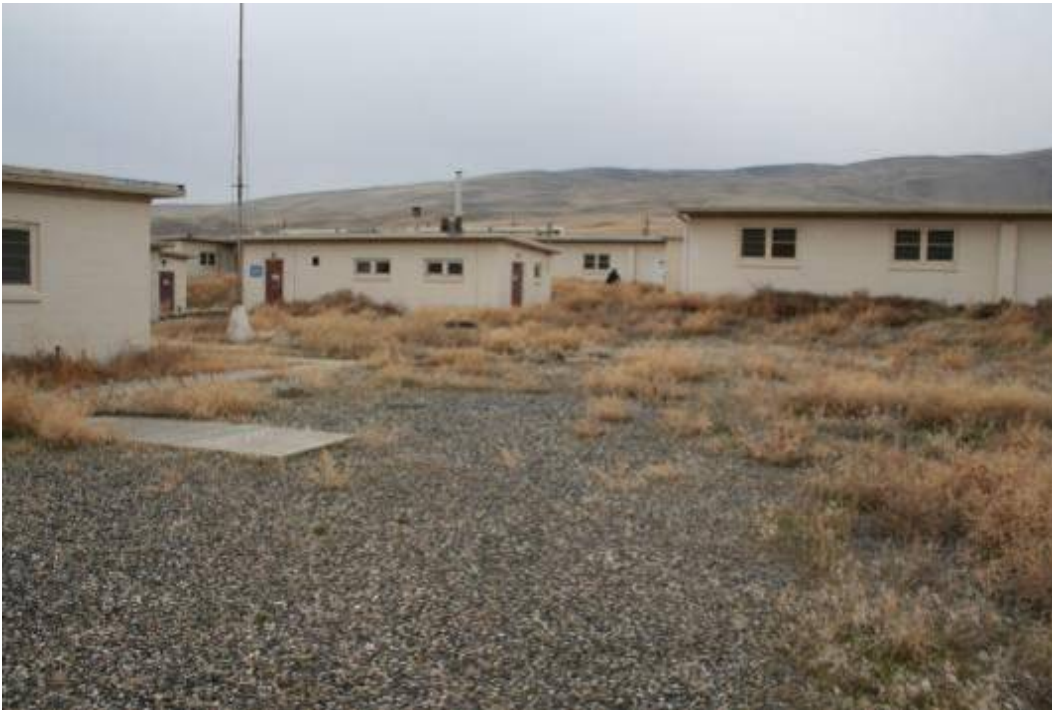
Figure A.38. Nike Offices (Base Area). Photo taken at 230 degrees on 3/19/09 by Doug McFarland.
