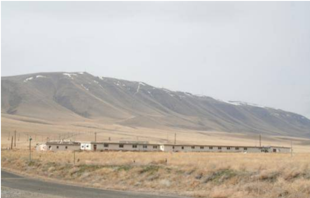
Figure A.35. Nike Buildings to Be Demolished. Photo taken at 280 degrees on 3/19/09 by Doug McFarland.
