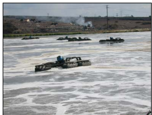
Aeration Lagoon at SABWWTP (Pond 1)
