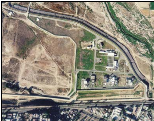
South Bay International Wastewater Treatment Plant
