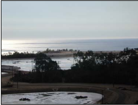
Lagoons at SABWWTP
