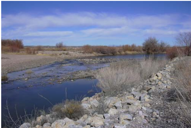
Photo 7. View of sediment accumulation at the Montoya Arroyo. Existing riprap protection on the east bank is shown in the foreground.
