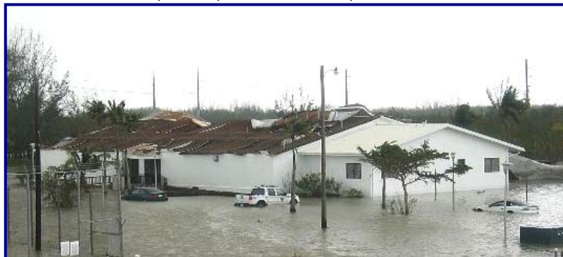
Naval Air Station Key West, FL is flooded after being hit by Hurricane Wilma.
