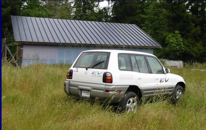
3.5 kW EV Charging Station
