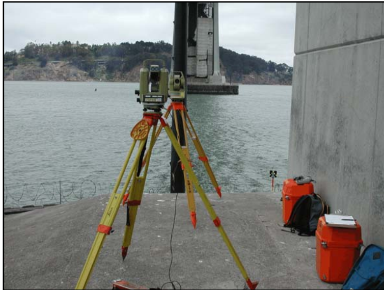
Figure 19. Total Station leveling operations on the San Francisco-Oakland Bay Bridge
