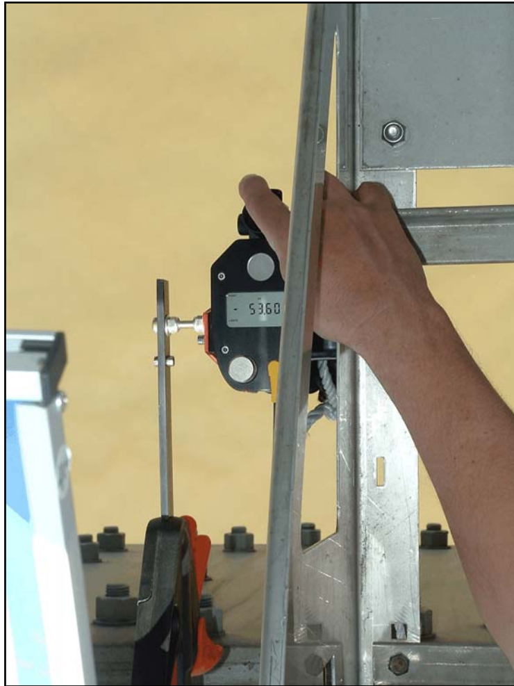
Figure 23. Laser range finder installed adjacent to microwave air gap sensor
