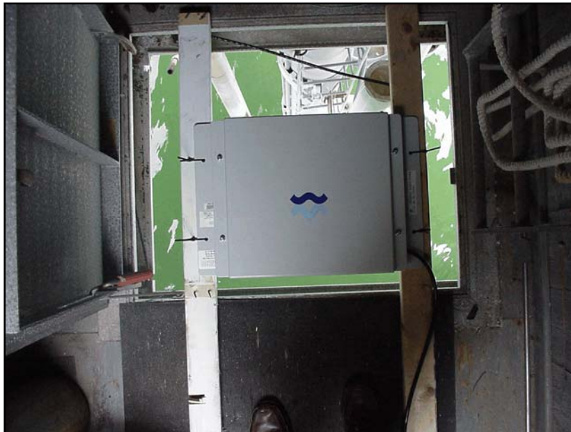
Figure 10. SM-094 temporarily mounted over the access hatch
