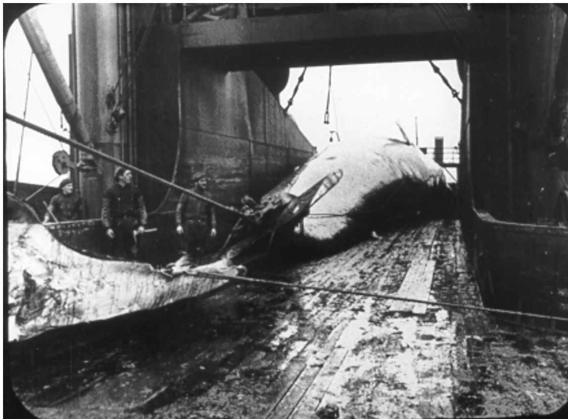
Fig. 12. "A whale arrives on the flensing deck. "A huge four ton claw is used to haul the whale up the slipway. This claw is so constructed that the greater the weight of the whale the tighter the jaws grip the flukes."
