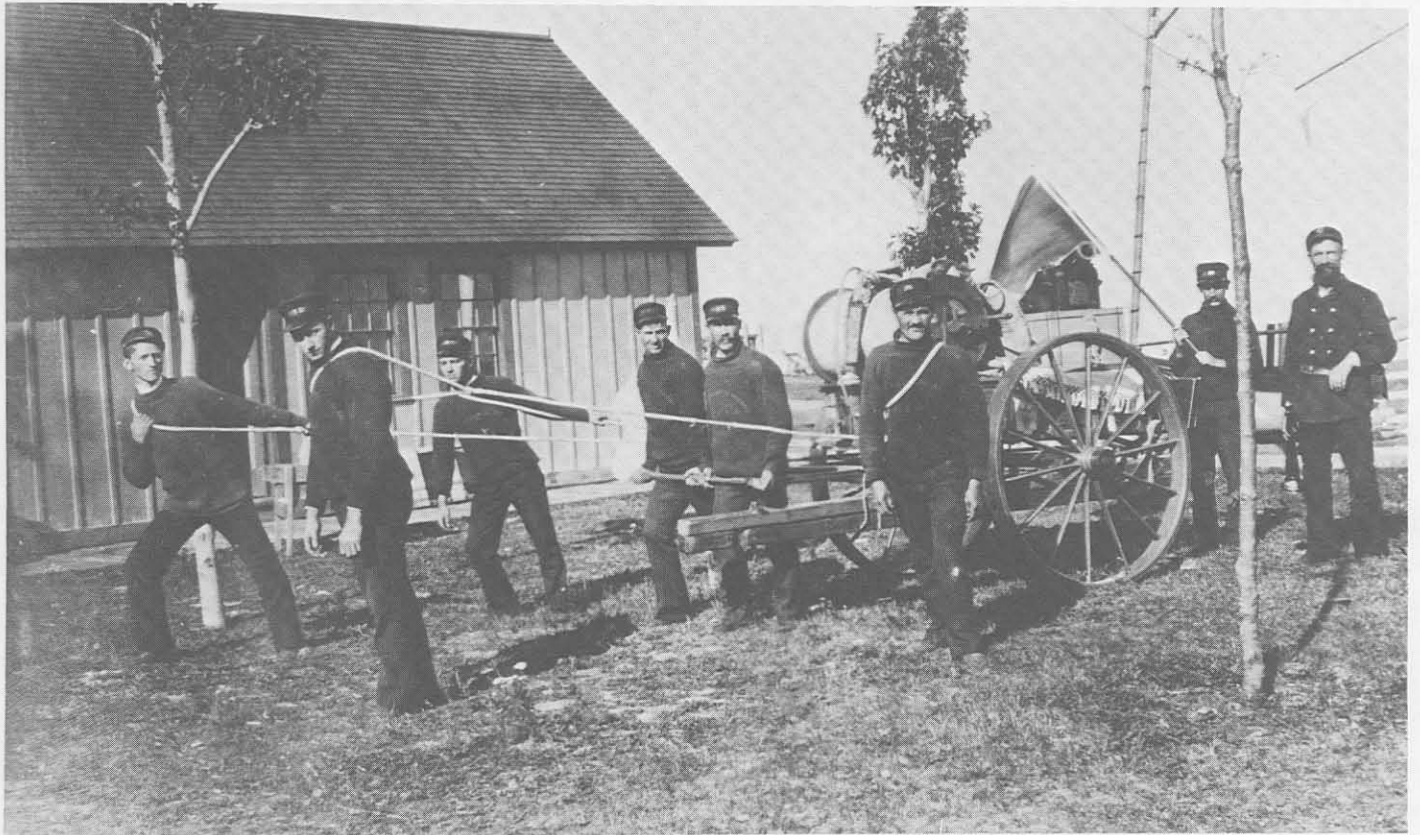
This beach cart is ready to travel. The Lyle gun can clearly be seen on top of the cart. Note the speaking trumpet in the right hand of the keeper at the extreme right. Pulling the cart through sand dunes could be very tedious.
