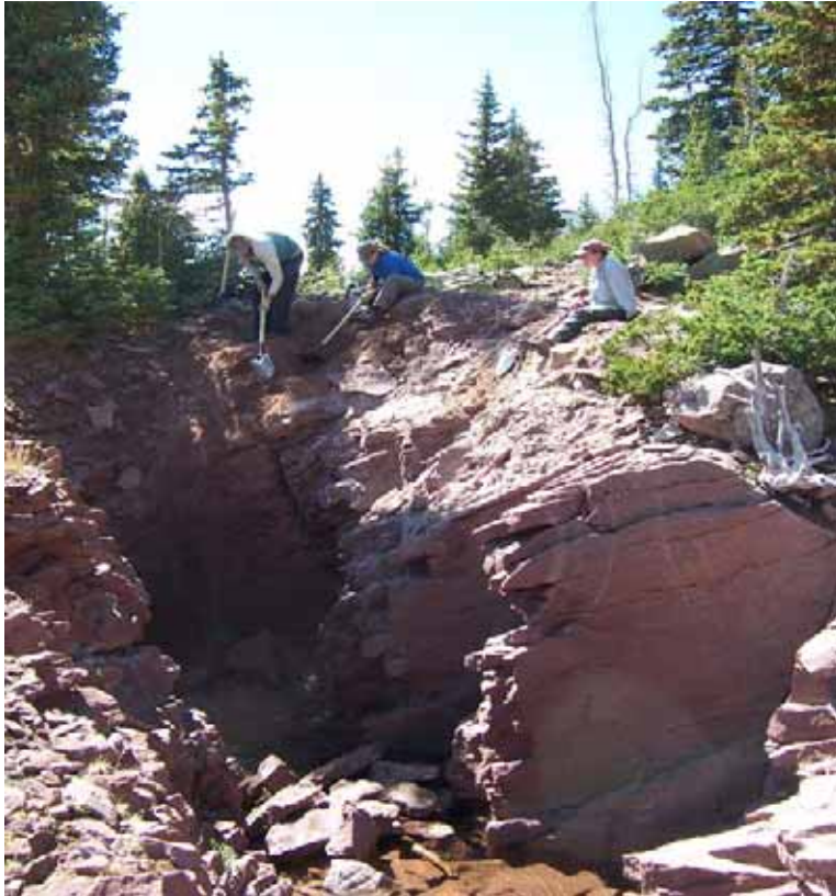
Figure 10. Crews pushing fill into inlet area.
