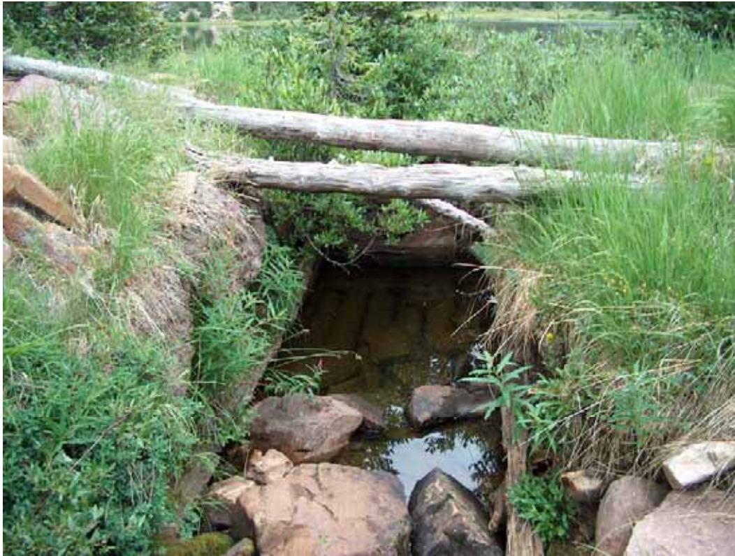
Figure 13. Pre-work outlet channel.
