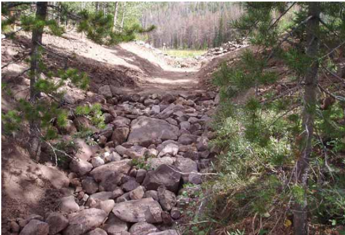
Figure 4: Excavated channel, looking upstream.
