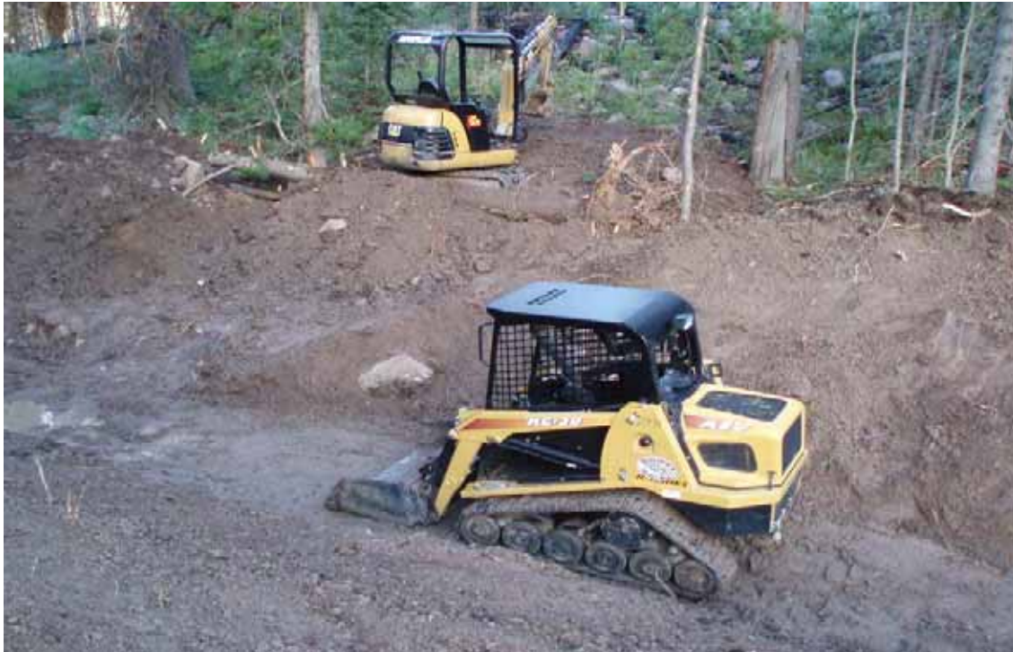
Figure 3: Excavation of the spillway.
