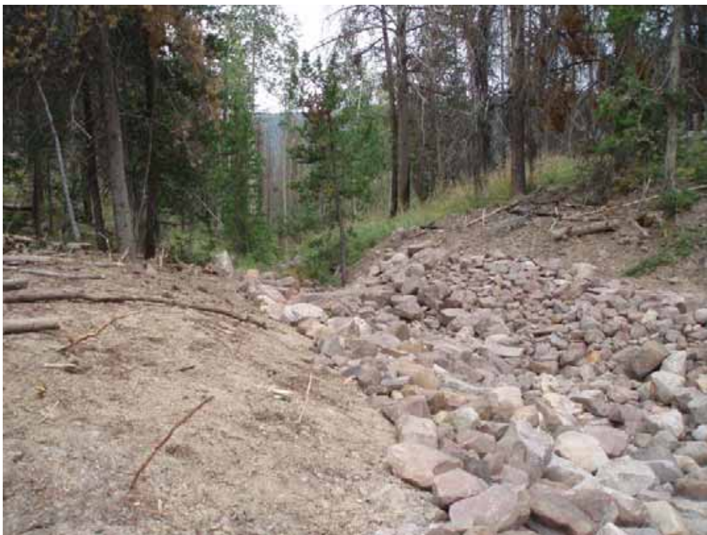
Figure 6. New spillway, looking downstream.
