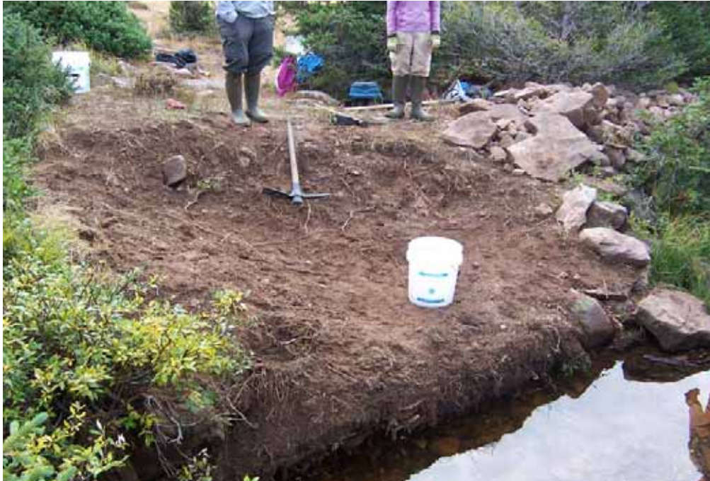
Figure 15. 2:1 slope on bank.
