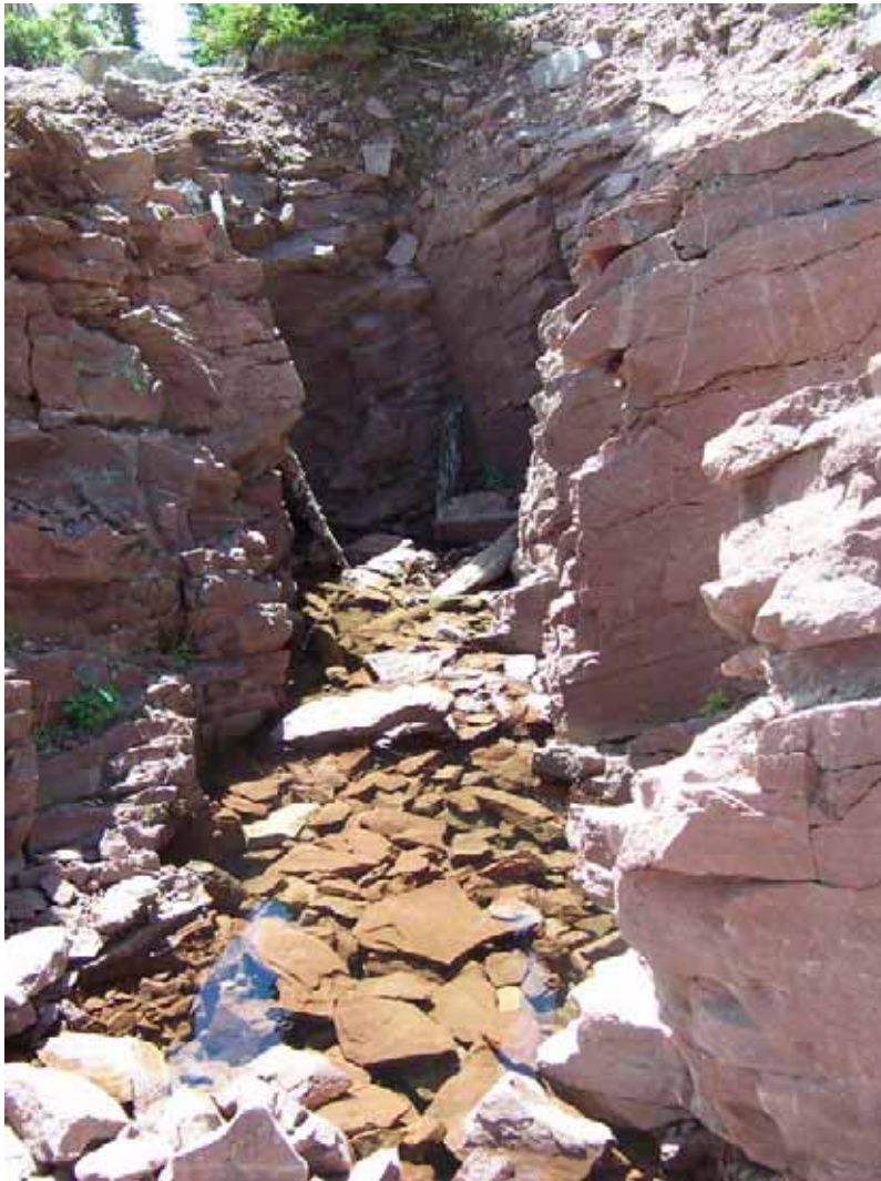
Figure 7. Upstream end of outlet tunnel.
