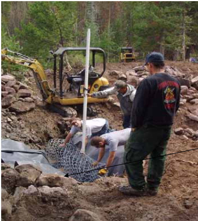
Figure 5. Preparing gabion basket wall.
