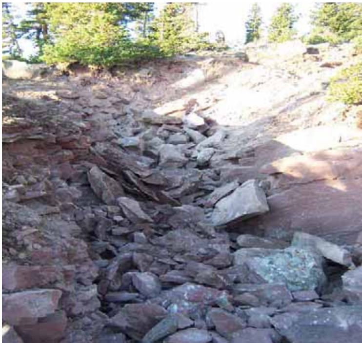
Figure 11. Finished inlet area.
