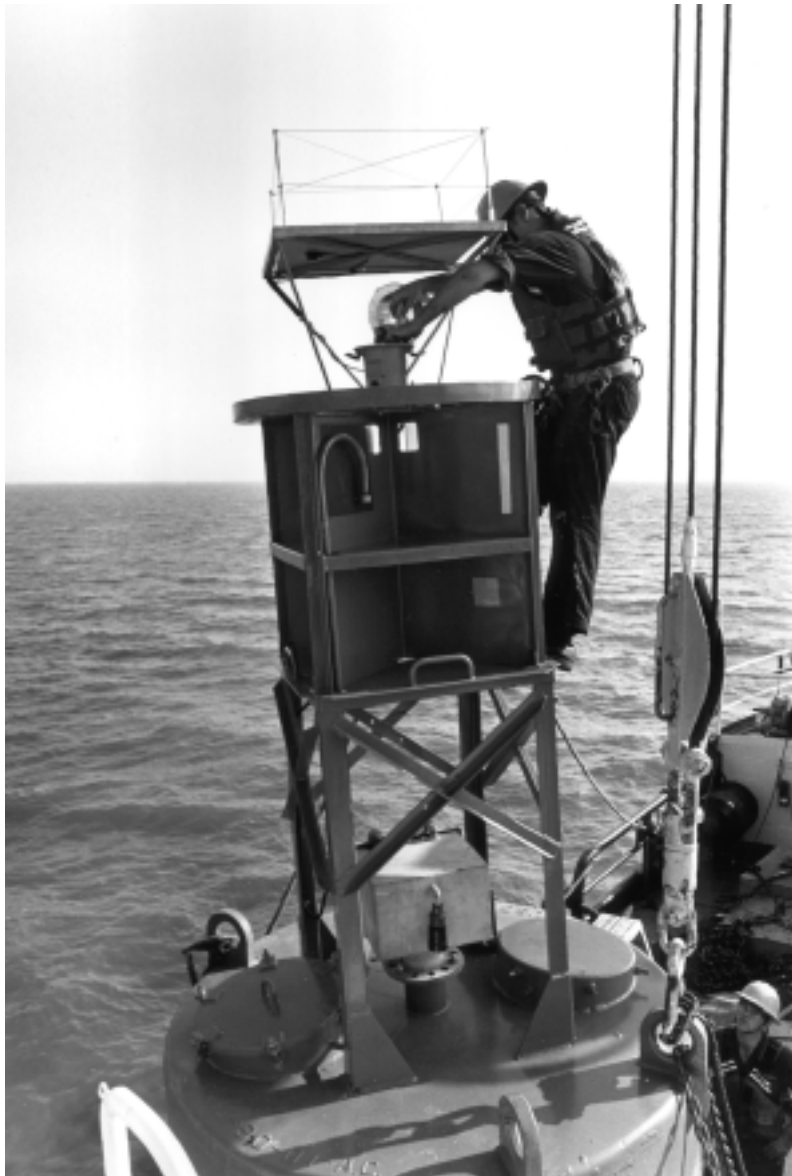
White Sumac crew member changes bulb on solar powered buoy (2001 HAER photo by Candace Clifford).
