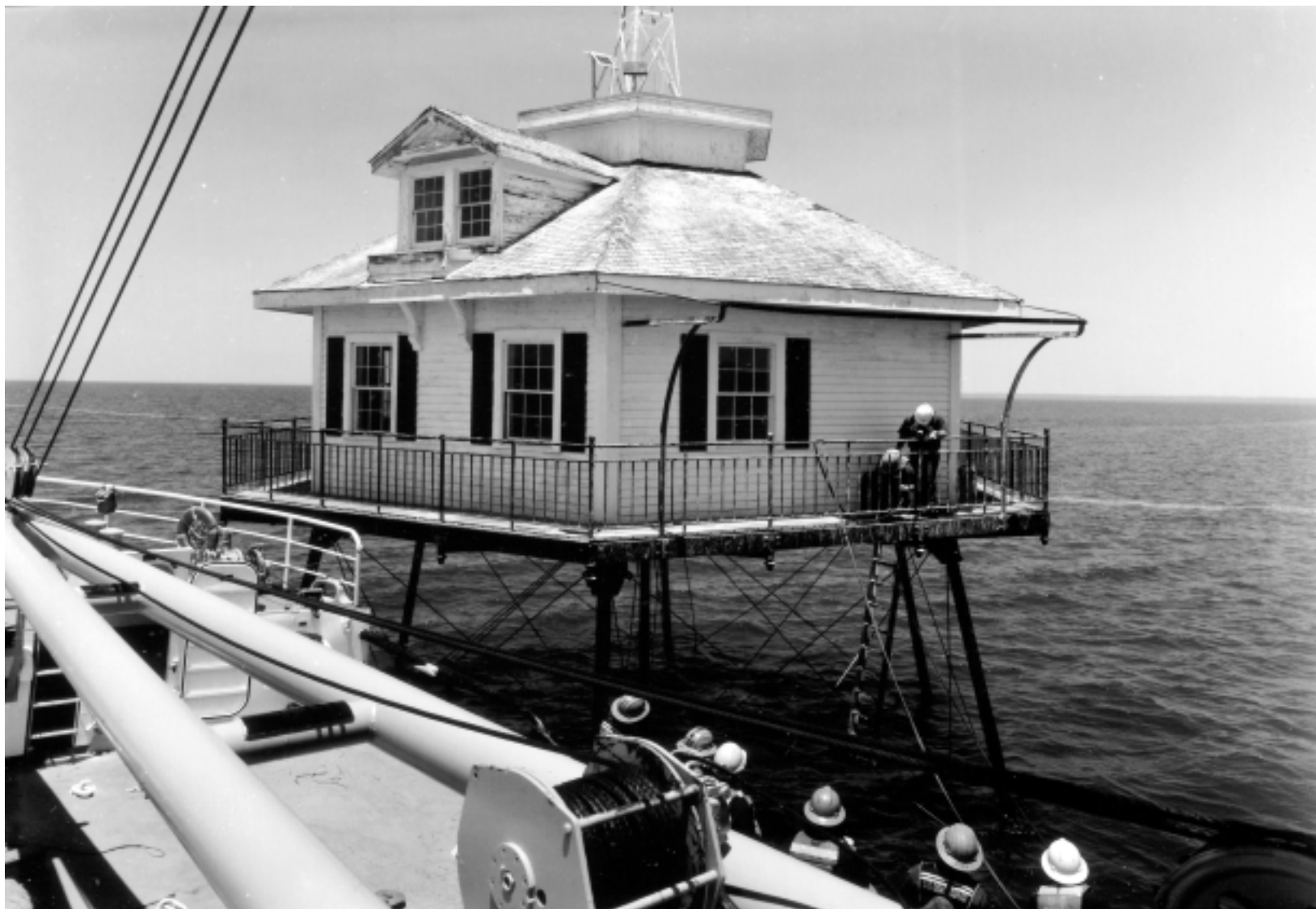
As part of maintenance, White Pine's crew removes rusty ladder for repair (1999 HAER photo).
