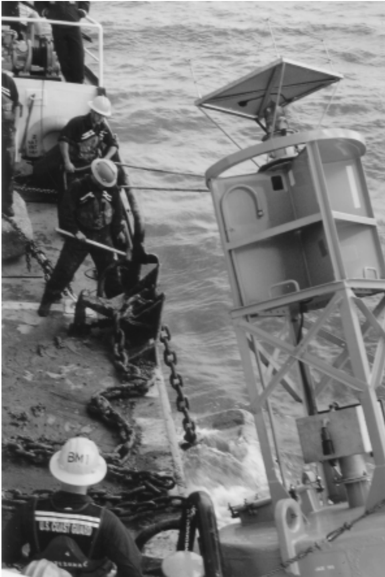
White Sumac crew prepare to release sinker and chain after maintenance of buoy (2001 HAER photo by Dana Lockett).
