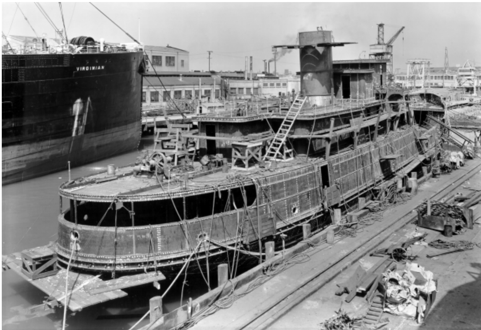
(Above) The framework in place, work on installing deck machinery and hardware begins. Photo taken April 1, 1939, courtesy of the Coast Guard Historian's Office. (Facing page) Detail of twin propellers taken while Fir is on the marine railway. Photo taken April 28, 1939, courtesy of the Coast Guard Historian's Office.
