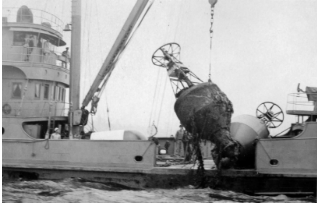
Servicing buoys aboard Fir in 1943: (Right) Bringing aboard a double bluff whistle buoy. (Below left) Scraping off sea growth. (Below right) Preparing scraped and repainted buoys for relief. Photos courtesy National Archives, Seattle.
