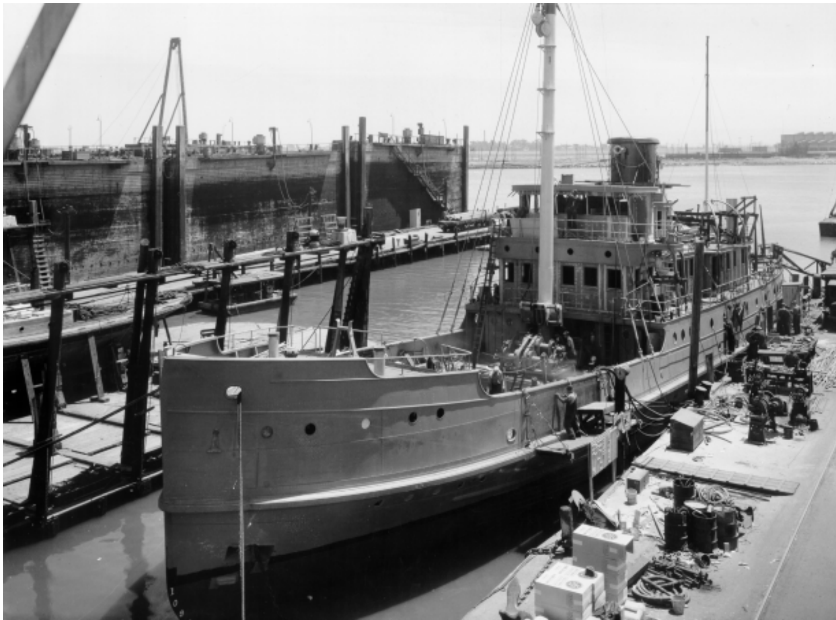
Nearing completion, Fir at the 'fitting out pier' on June 30, 1939. Photo courtesy of the Coast Guard Historian's Office.
