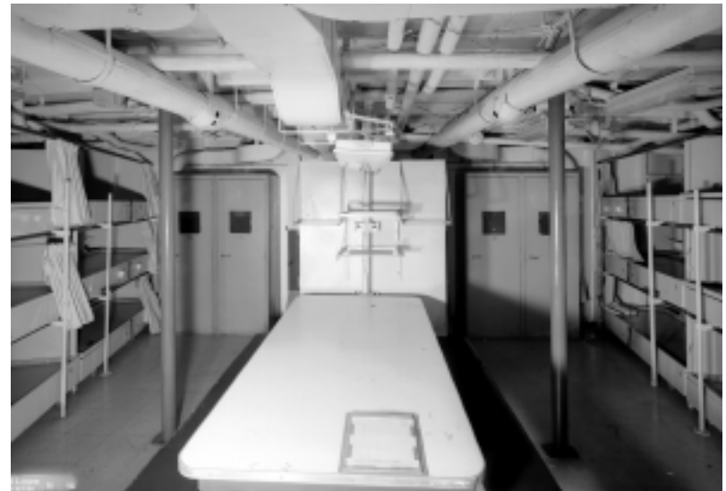
Detail of Fir's hoisting boom (above) and berthing (below) in 2000. HABS/HAER photos by Jet Lowe.
