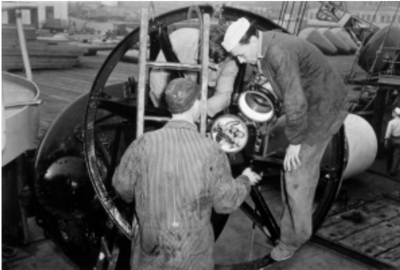
Lamp changer and mechanism are being completely checked and tested after being reattached to renewed buoy before it is taken off the dock. 1943 photos courtesy of National Archives, Seattle.
