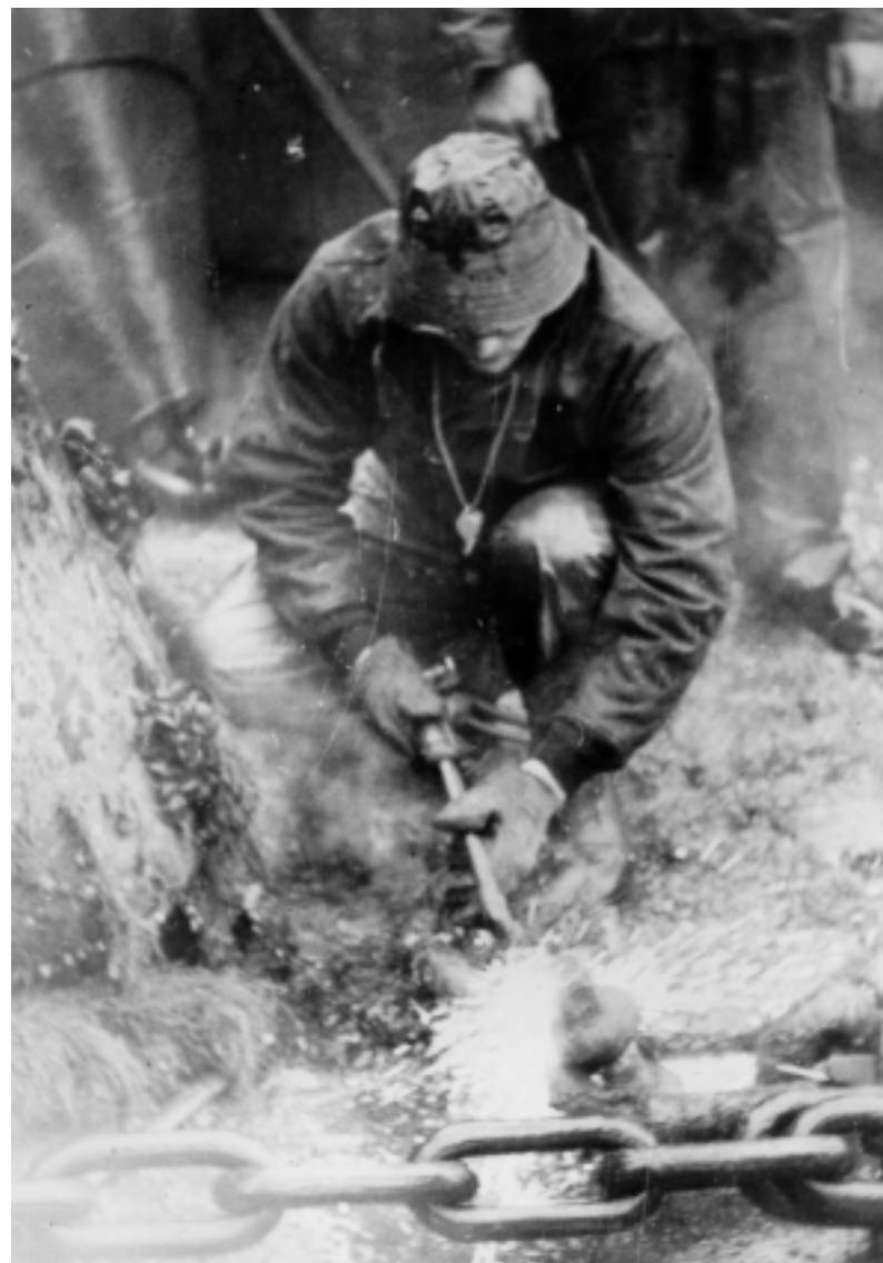
Fir crewman alters buoy mooring chain. Photo courtesy National Archives, Seattle.
