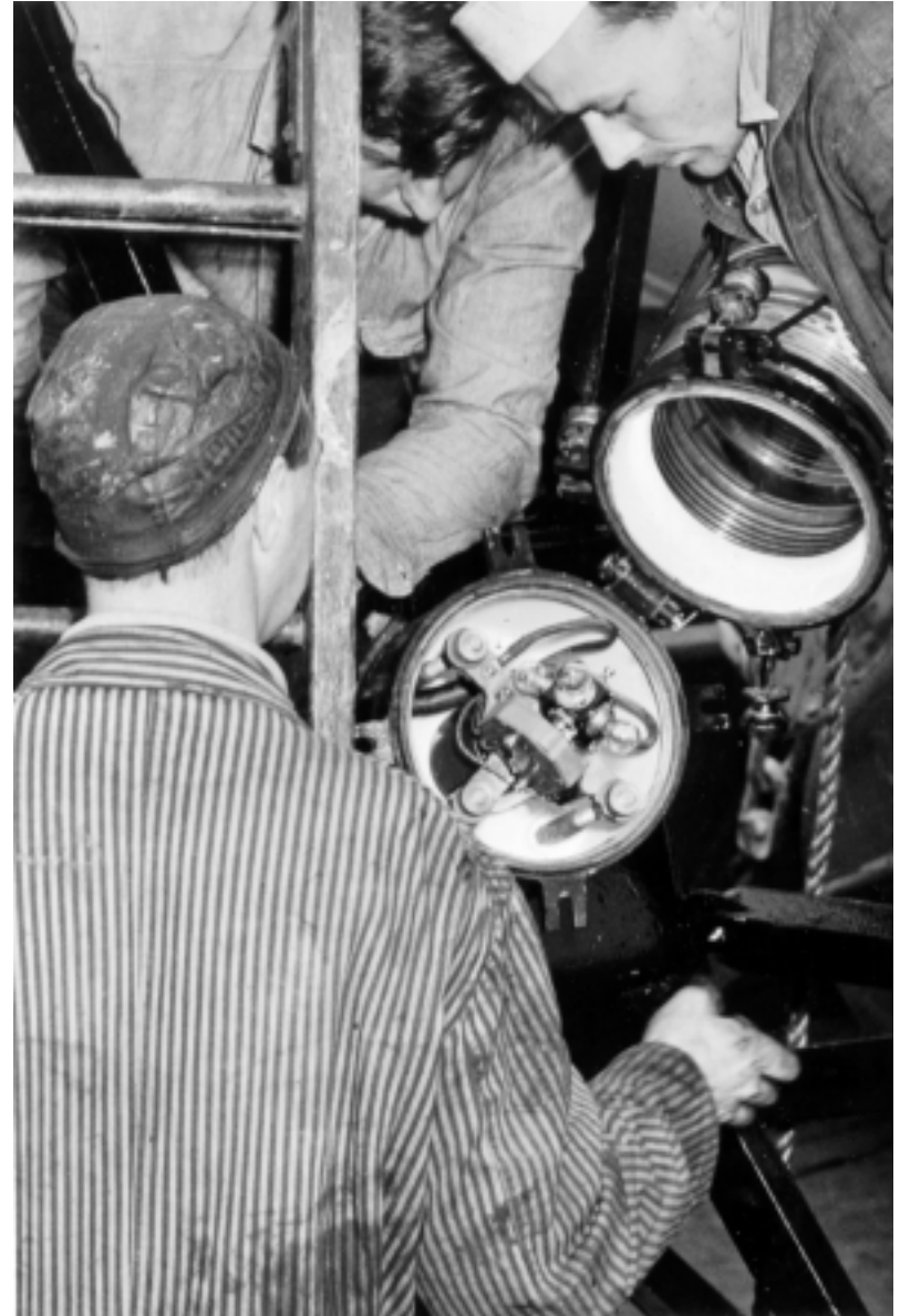
Lamp changer and mechanism are being completely checked and tested after being reattached to renewed buoy before it is taken off the dock. 1943 photos courtesy of National Archives, Seattle.
