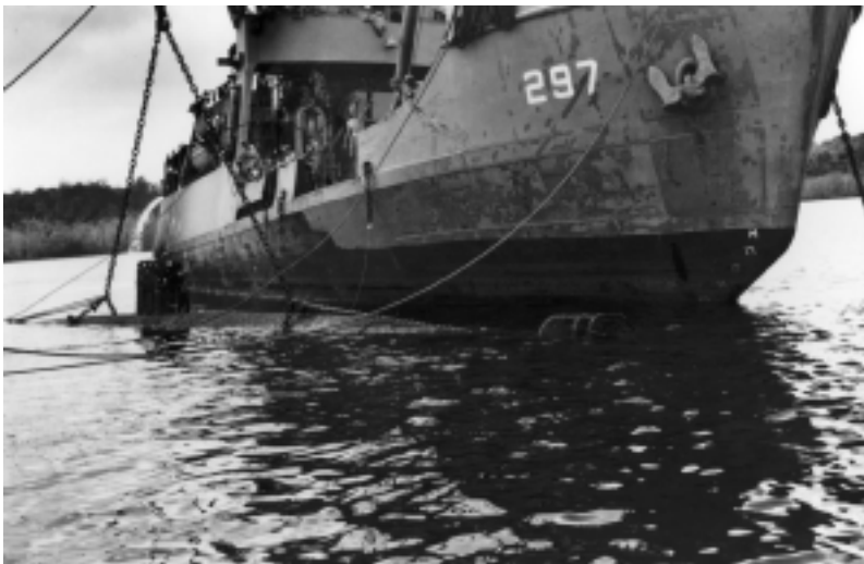
Ironwood salvages a Japanese midget submarine in the South Pacific during World War II. The heavy lift capacity of buoy tenders was regularly used in salvage operations throughout their careers.
