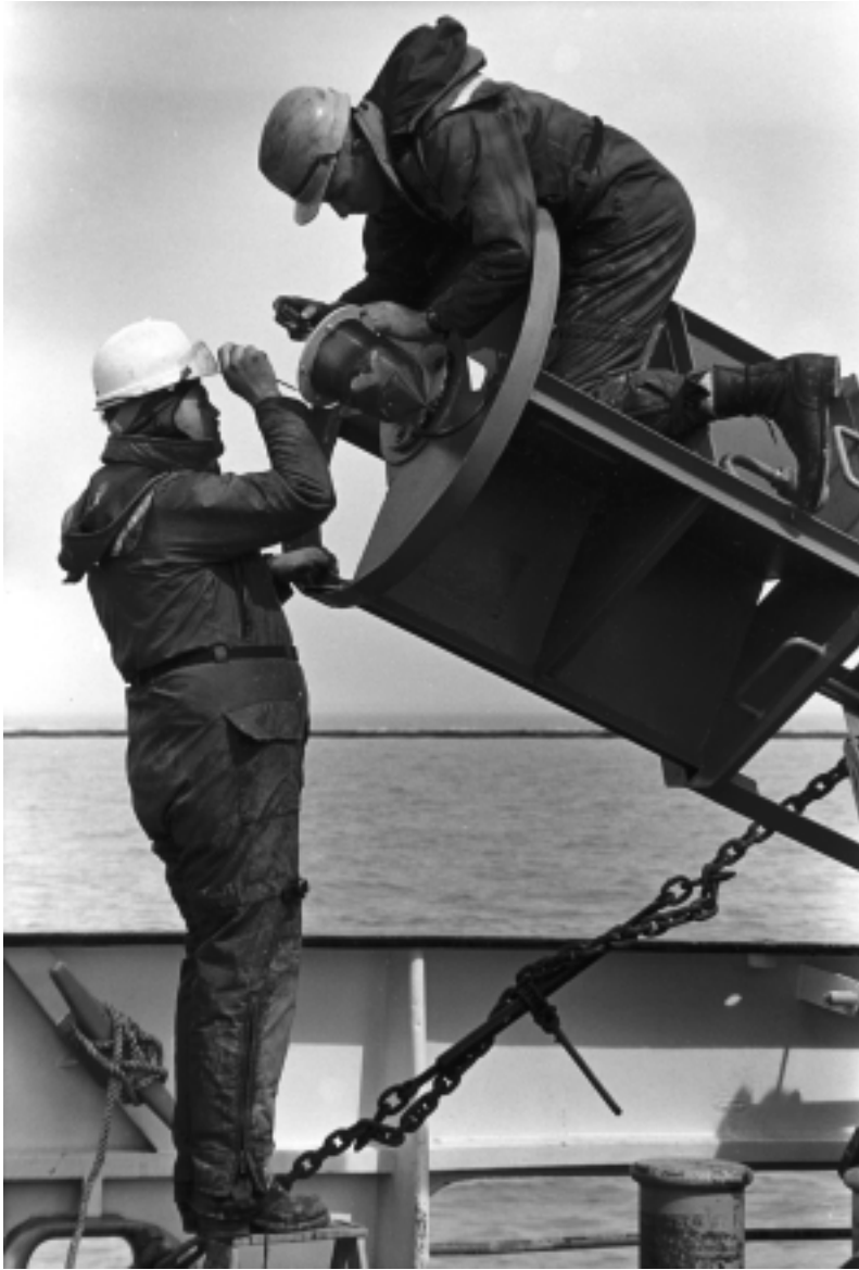
Two members of a buoy tender's deck force service a light on a navigational buoy.
