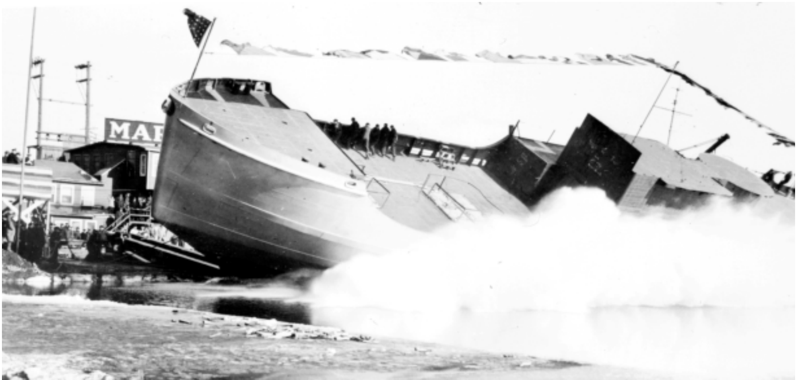
The finished hull of a 180 is launched in Duluth, Minnesota. Note the men holding onto the rail and riding the vessel during its launch.
