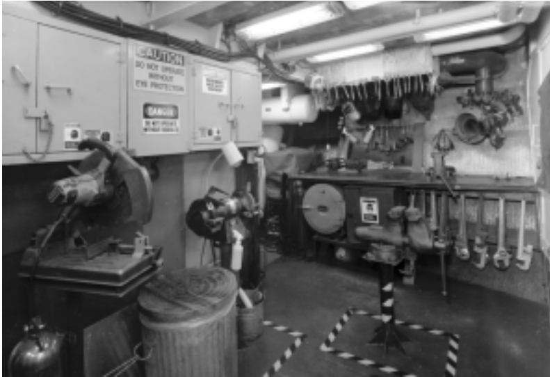
Damage control shop which was added aboard Sundew during renovations. HABS/HAER photo by Jet Lowe.
