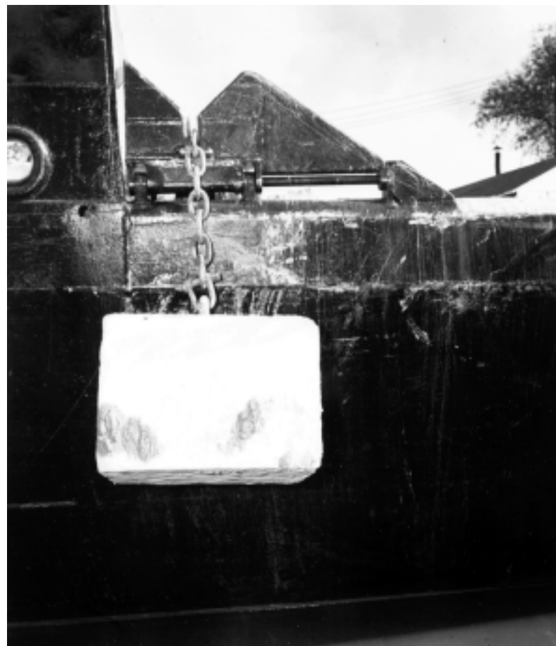
(Facing page) A buoy is loaded onto Buttonwood in preparation for a buoy tending mission. Note the bridge-mounted vang system for the boom and the post-war color scheme. HABS/HAER photo by Jet Lowe. (Above) An outboard view of a sinker suspended over a buoy's side through a chain stopper.
