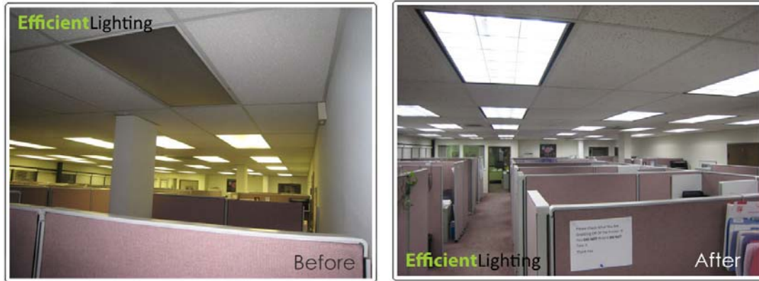
Figure C.4 Example of Improved Lighting Appearance with Energy Saving Lighting Retrofits (Efficient Lighting, 2008)
