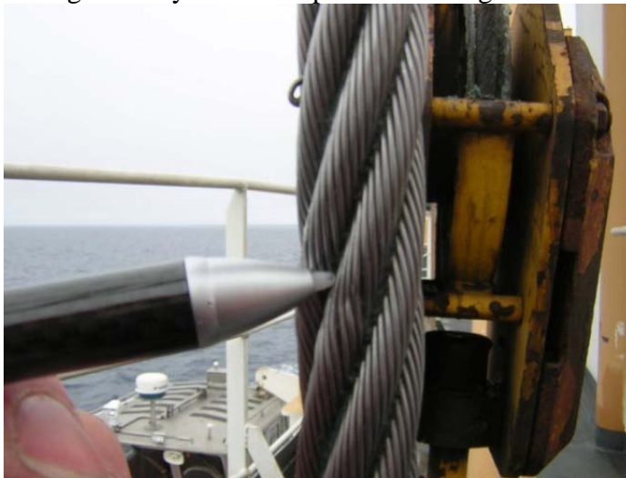
Kink in 04 Deck Crane cable
