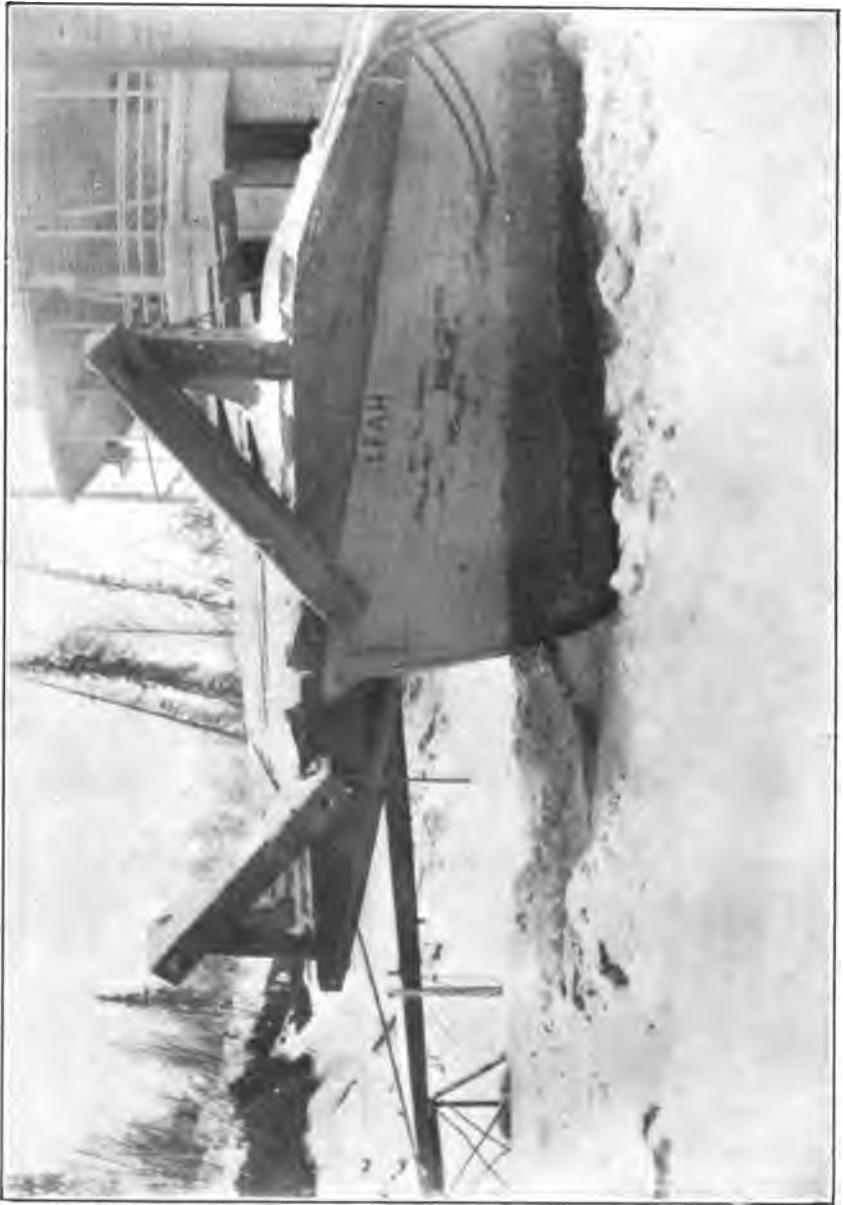
METHOD OF CONSTRUCTING THE BOW OF YUKON RIVER STEAMERS USED IN TOWING BARGES, LASHED AHEAD.
