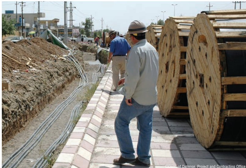
Iraqi workers on an IRRF project inspect recently dug cable trenches to ensure underground power cables have been laid correctly. Improved electrical services for local Iraqi homes and businesses will decrease dependency on neighborhood generators and provide a more continuous supply of power for local residents.
