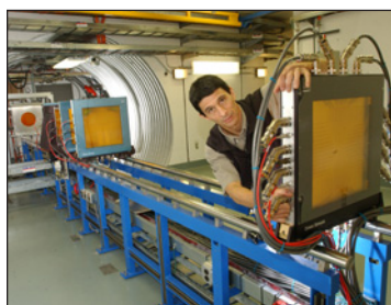
Inside the target room of the NSRL are four ion chambers used for beam imaging (black-framed objects) or dosimetry (blue-framed objects).
