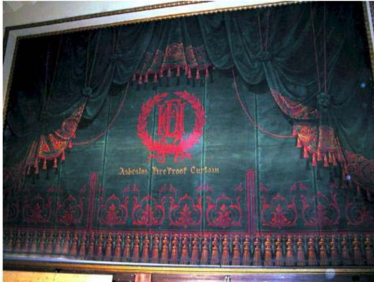
Asbestos Fire Curtain – Removed and Stored for Future Display. There was no existing documentation regarding the fire curtain, so we didn't know it was so elegant!
