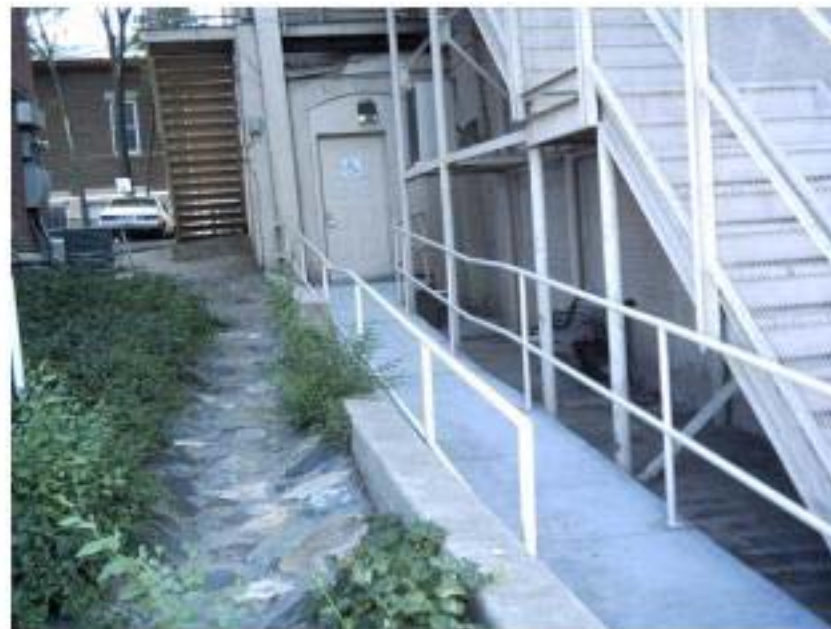
Right: After Renovations
