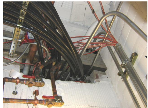
Picture 5 Penetration in a fire wall
