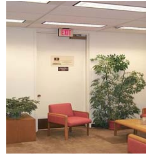
Blocked exit route
