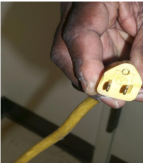
Appliance plug missing ground prong
