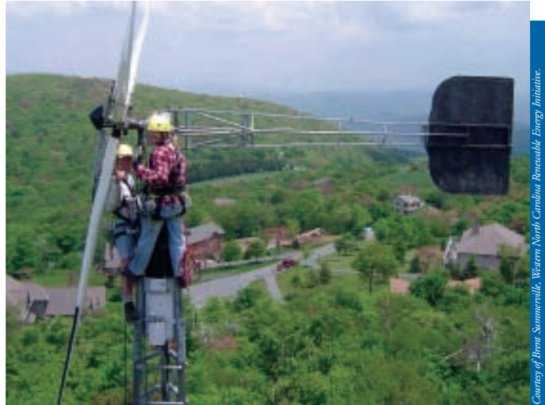
Repairmen at the North Carolina Small Wind Initiative's research and demonstration site on Beech Mountain.
