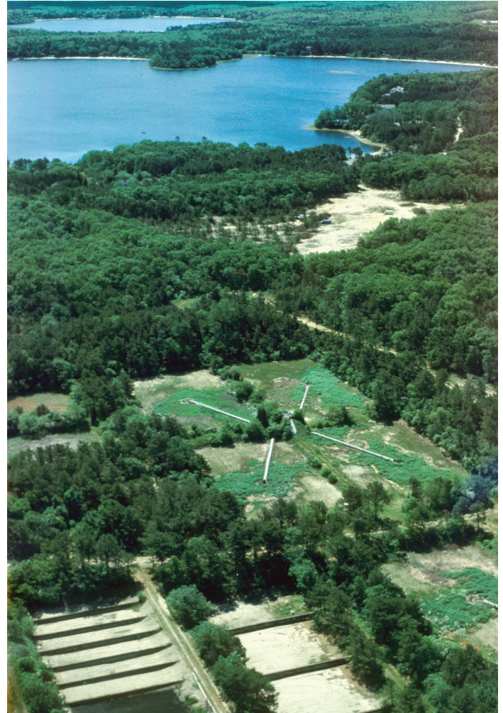
Southeast view of wastewater-disposal beds and Ashmet Pond
