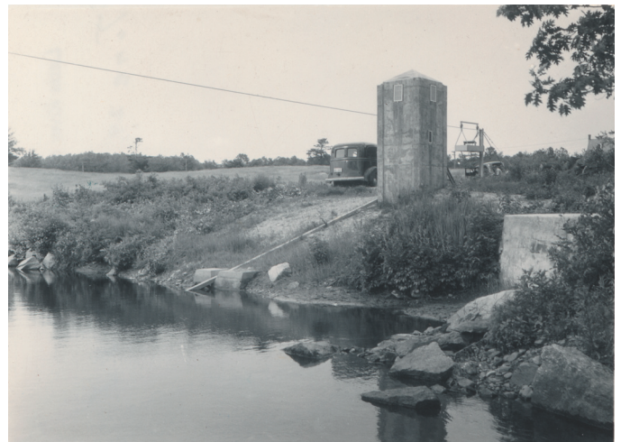
Streamflow-gaging station Little River at Oxford, Massachusetts. This 1940 photo shows the gage house, cable car, and cableway.
