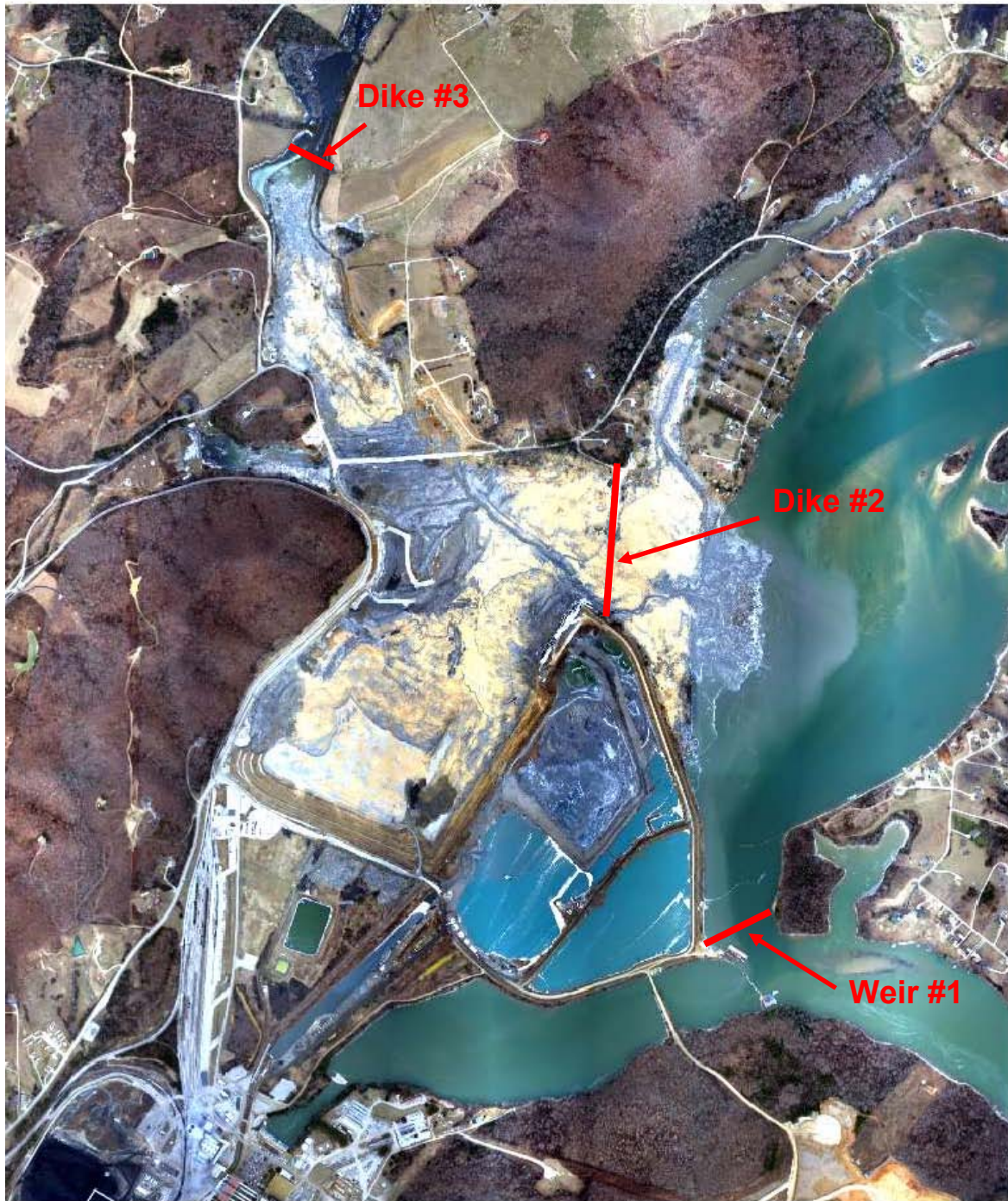
Aerial Image of Kingston Ash Slide 01/17/2009
