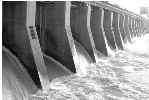
Spills occur more often at main-river dams because these projects manage the bulk of the water flowing through the system. Your best bet for seeing a spillway in action is at Kentucky Dam, where spillway releases occur on average more than 100 days a year. Contrast that to Norris Dam, where the spillways have been used only in nine of the 67 years the dam has been in operation.
