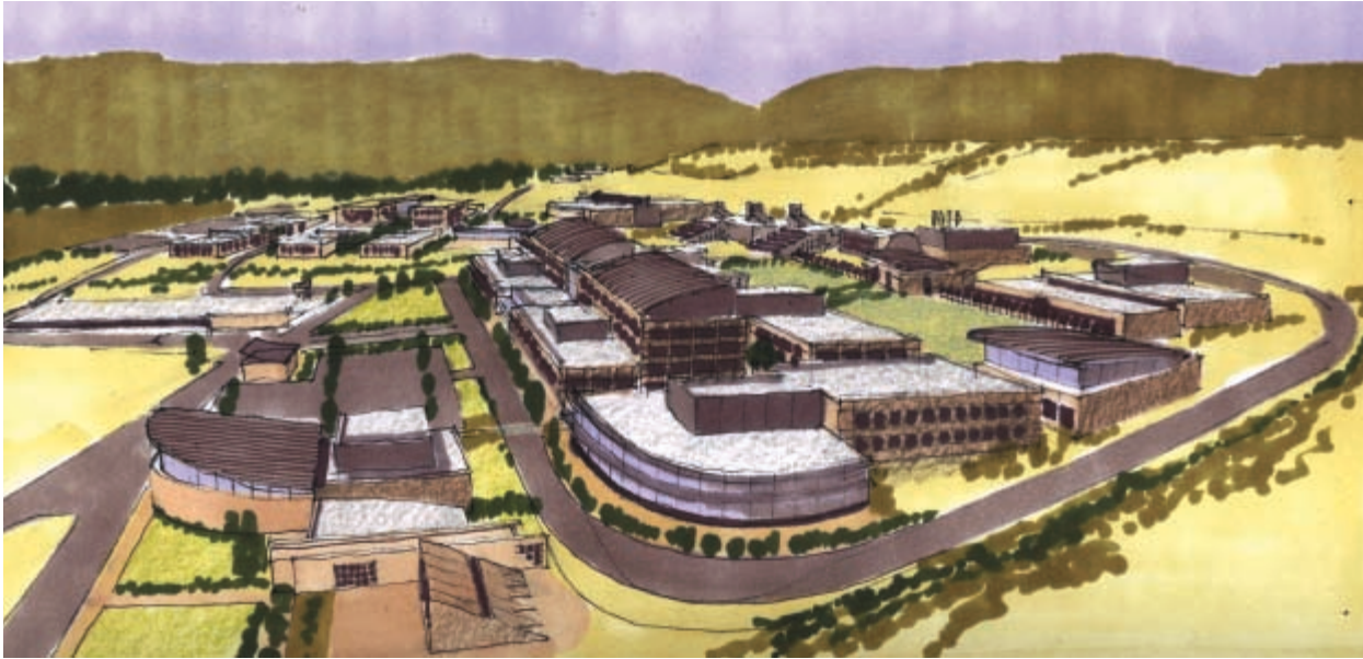
Figure 3-3. View from the East End of the Campus Looking West
