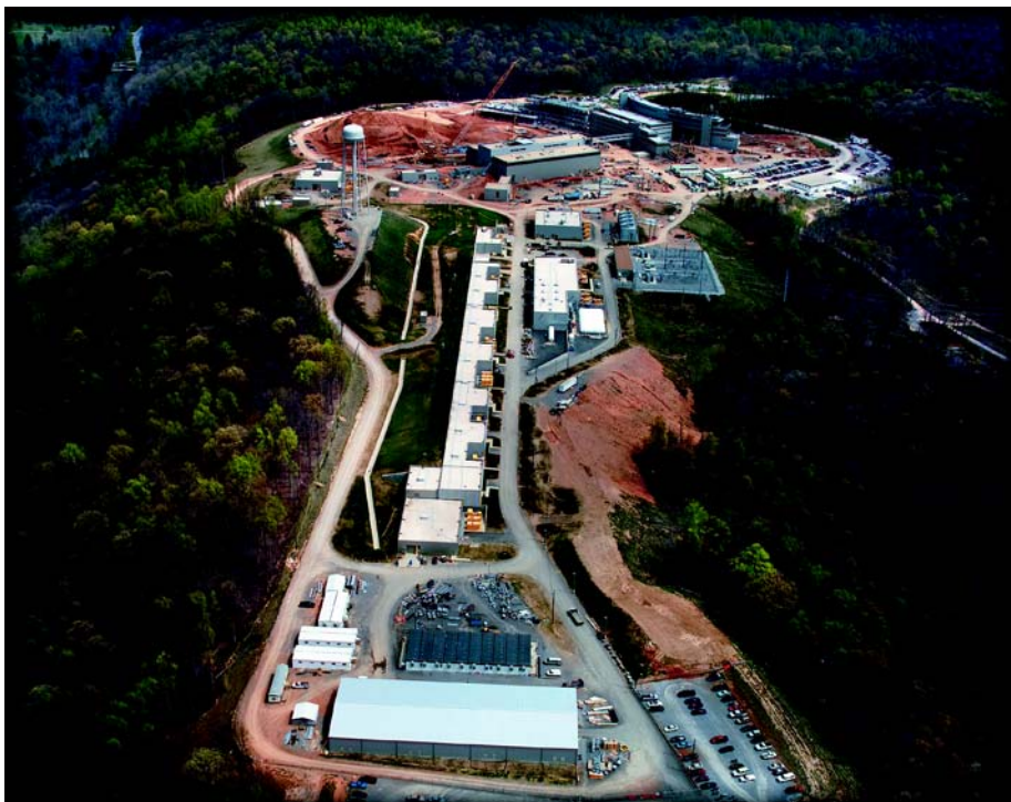
Eastward view of the SNS site, April 7, 2004. The Klystron Building is prominent in the center, running the length of the underground linear accelerator tunnel. For more SNS photos, see the SNS Photo Gallery at web.ornl.gov/sci/iris/search_sns.shtml .
