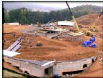
Construction on the ring tunnel.
