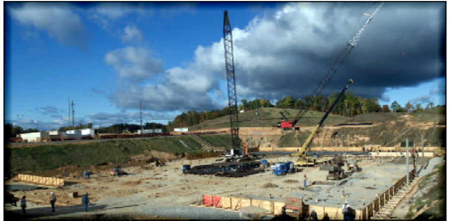
Construction at the target building foundation.
