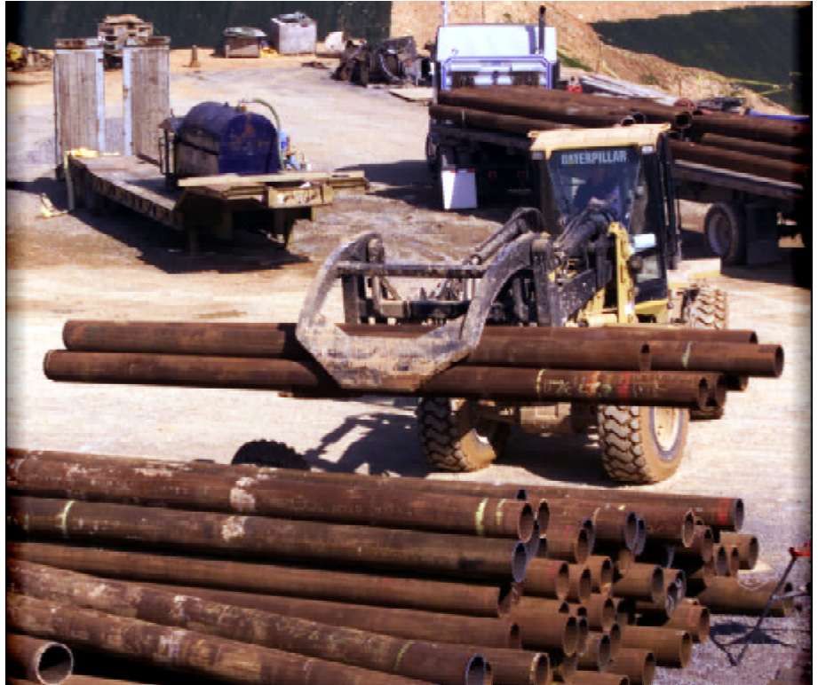
Staging material for the target facility’s mini-pile deep foundation.
