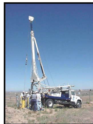
Installation of the Pneumatic Packer into a monitoring well
