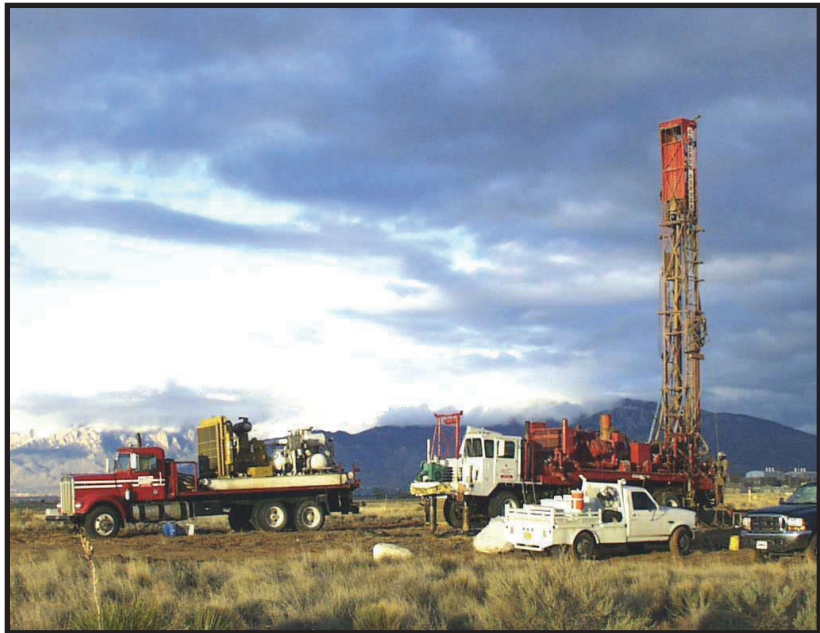
Mixed Waste Landfill Drilling Operations
