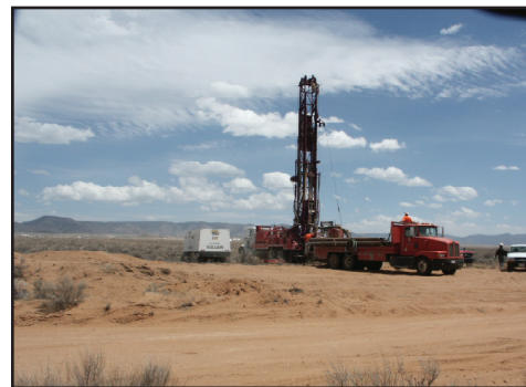
Drilling Operations at SNL/NM
