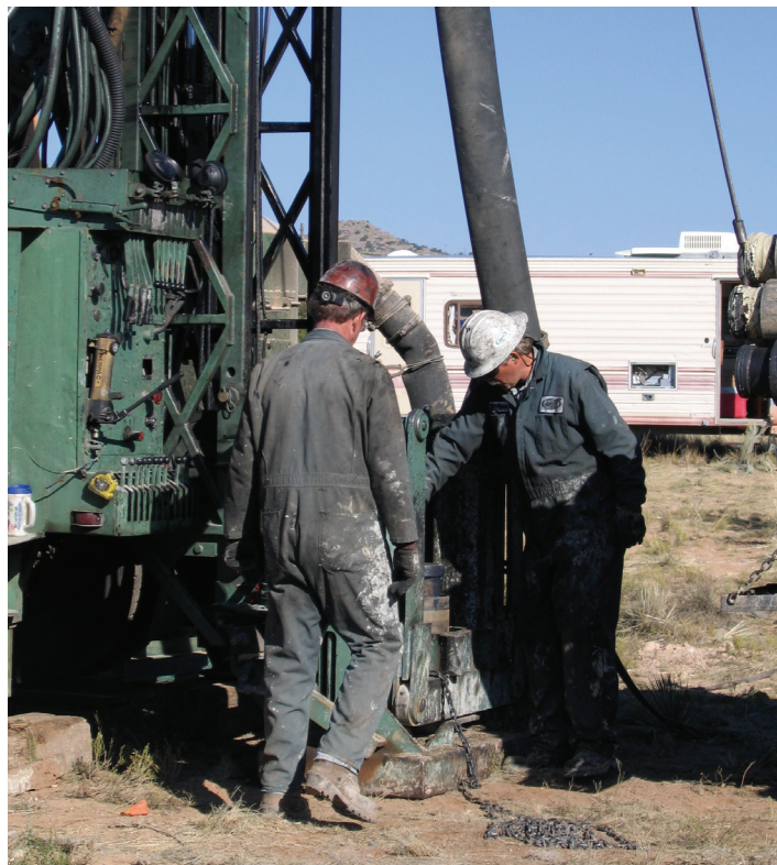
Groundwater Well Installation at SNL/NM
