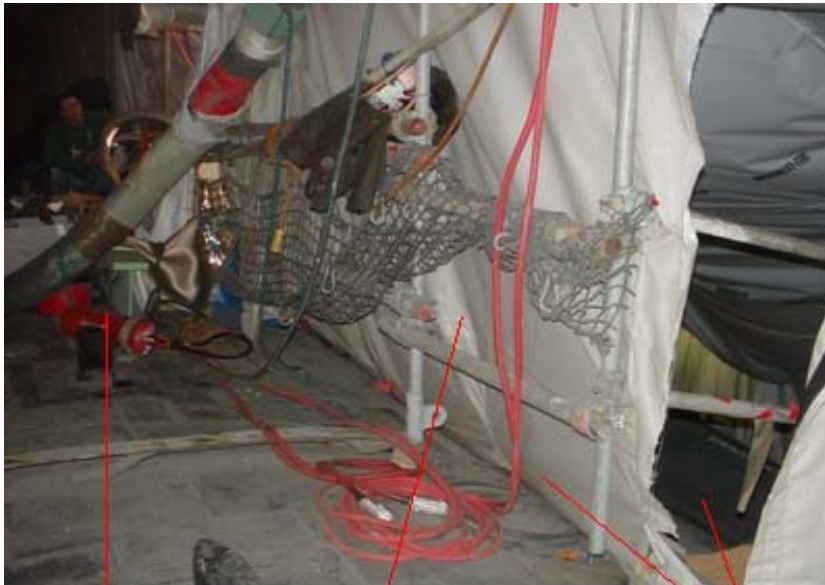
Netting not replaced following work
