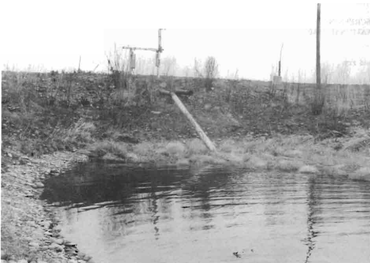
Figure 25.—(Above) Aerial view of water withdrawal site of W. Ketchersid. (Below) Example of a metal pipe straining device with slashes cut with a welding torch.
