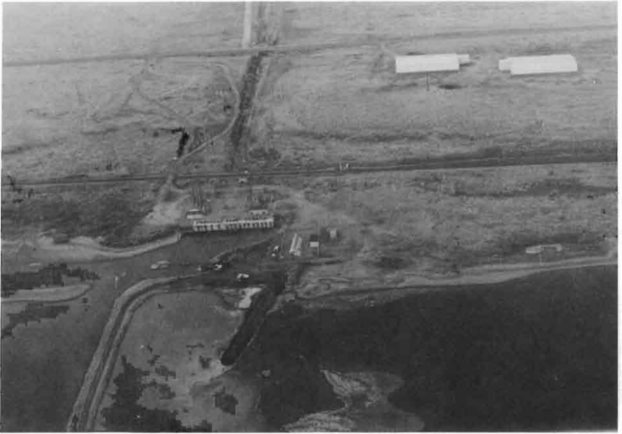
Figure 12.—Aerial view of Lorin Munn's water withdrawal site showing single, large, screened intake pipe.
