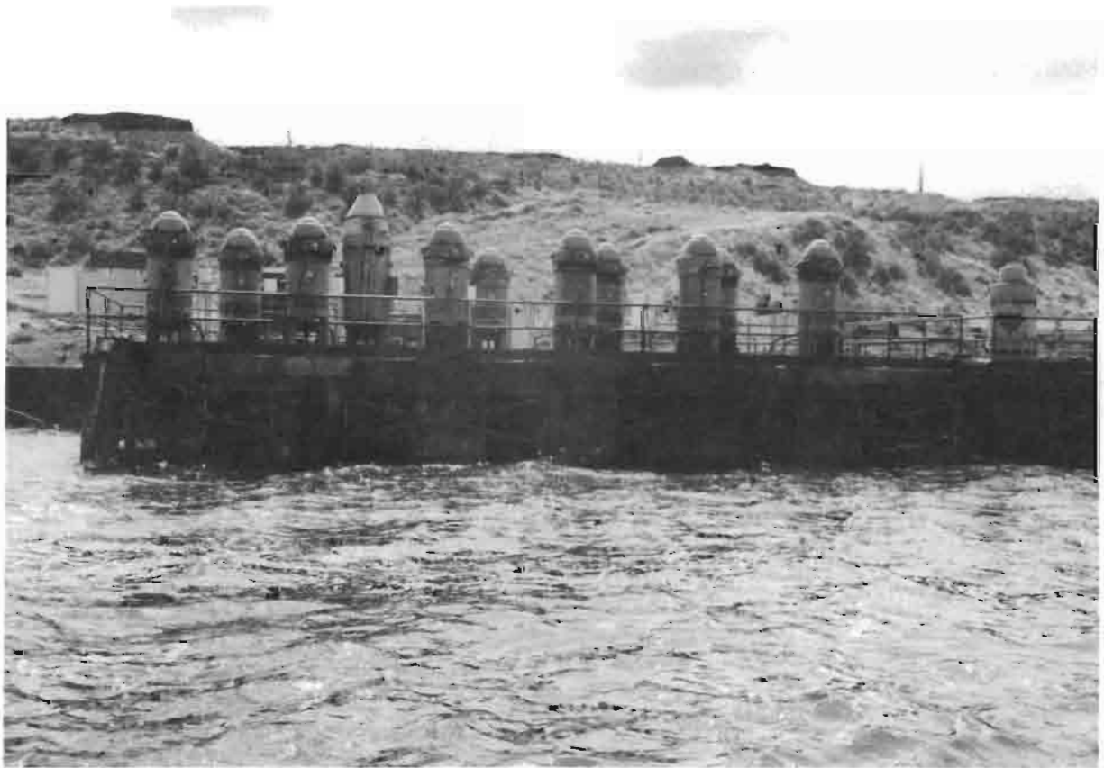
Figure 8.—(Above) Aerial view of water withdrawal site of Mikami Brothers. (Below) View of the pier-like water withdrawal structure out from the shoreline supporting turbine pumps.
