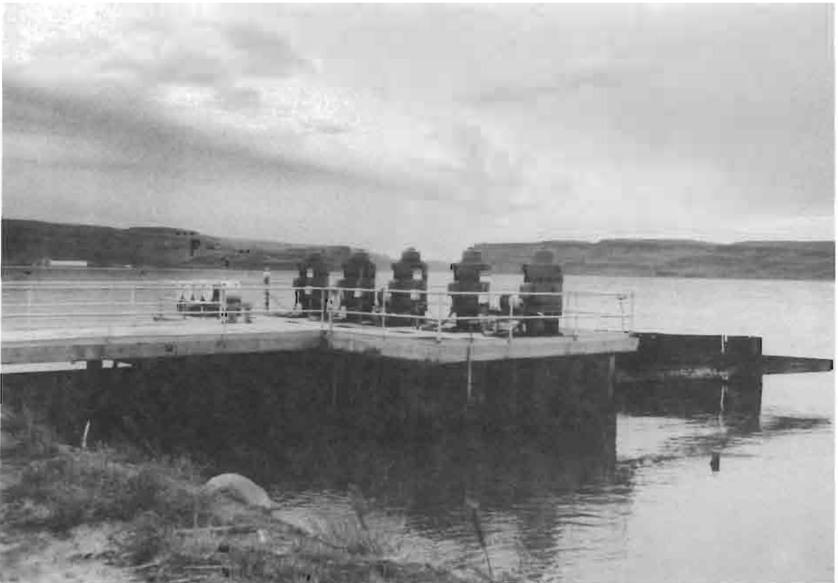
Figure 10.—Views of Nedrow Farms' combination pier/vault created by enclosing the area under a pier with driven sheet piling or other material.
