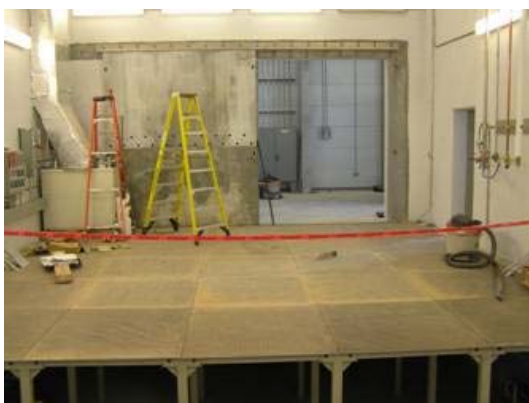
The shield doors and the suspended floor were installed.
