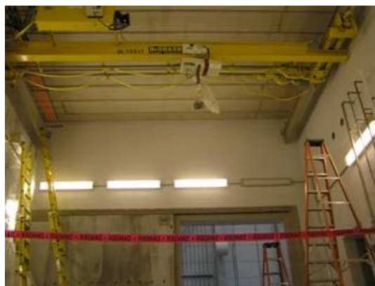
The VULCAN cave roof was completed.
