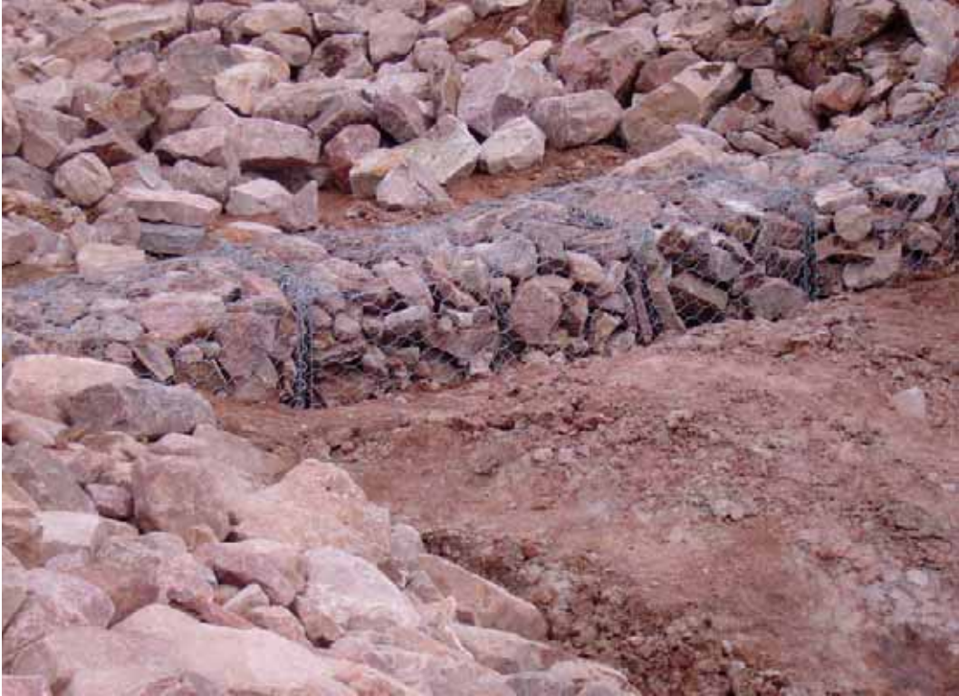
Figure 20 – Rock filled gabion baskets.
