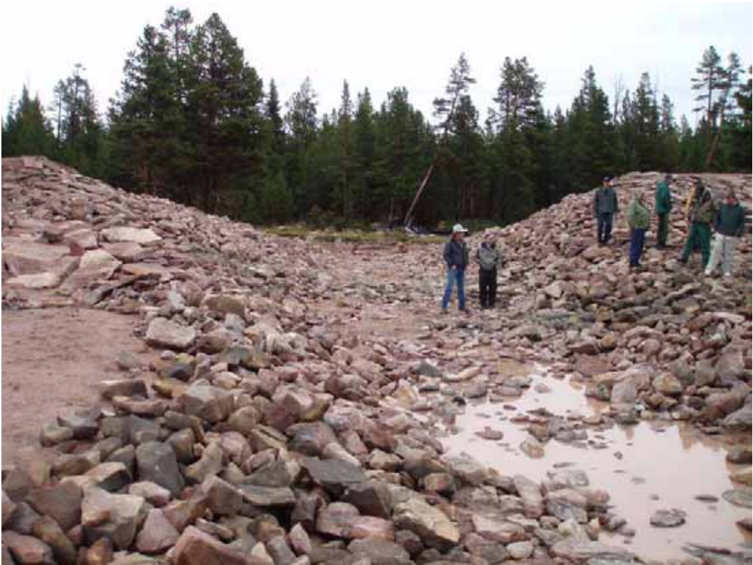
Figure 27 - View of group discussing the completed stabilized breach through dam embankment.
