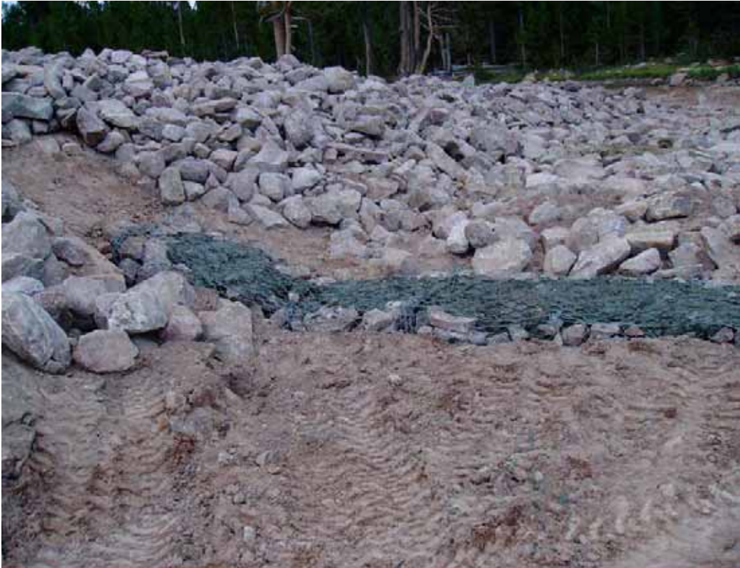
Figure 21 - Gabion baskets after grouting voids.
