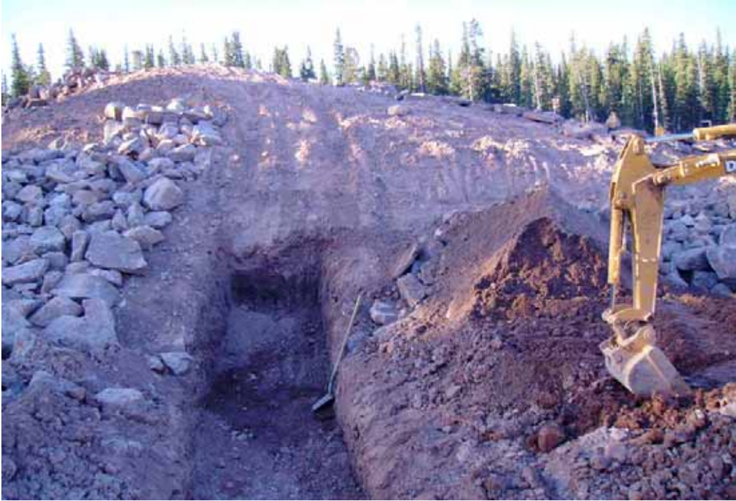
Figure 17 - Excavating middle cutoff trench.
