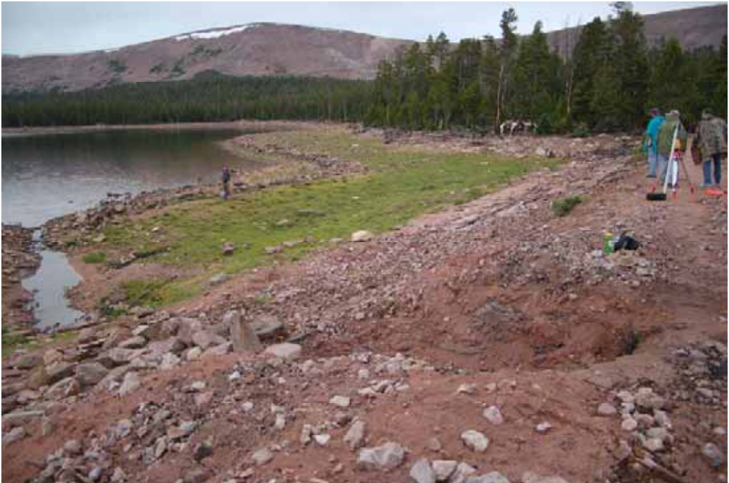
Figure 11- – View of dam embankment prior to arrival of equipment.
