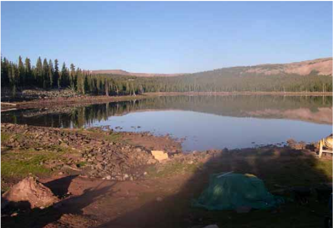
Figure 13 - Dam inlet and upstream face of dam at the start of work.
