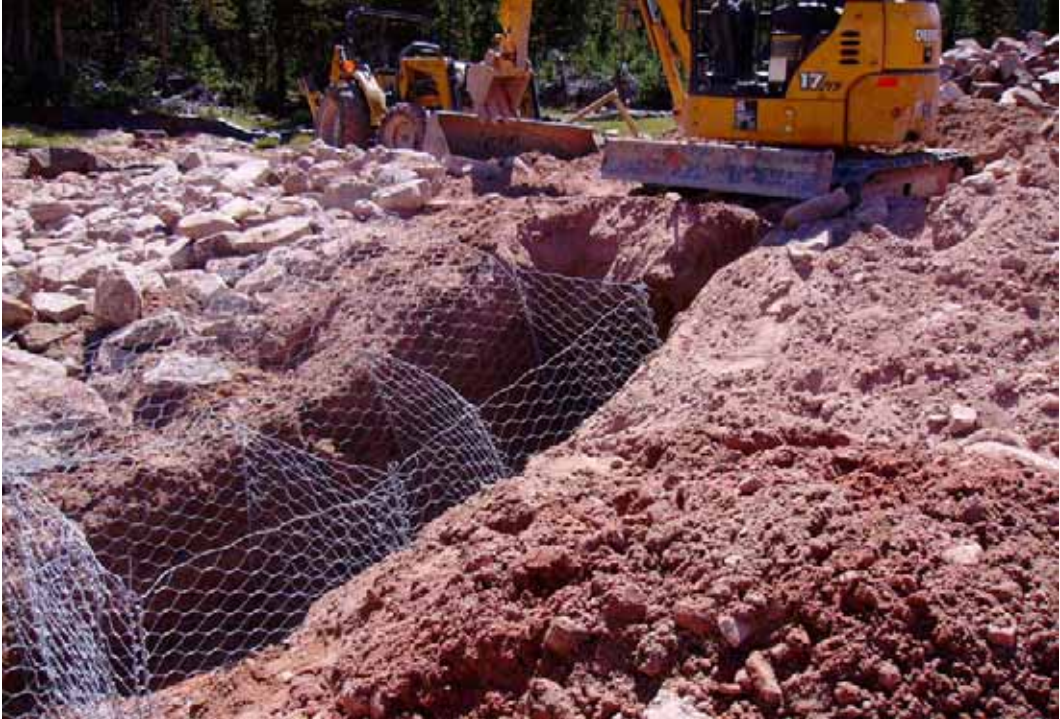
Figure 18 - Installation of the downstream gabion basket cutoffs.
