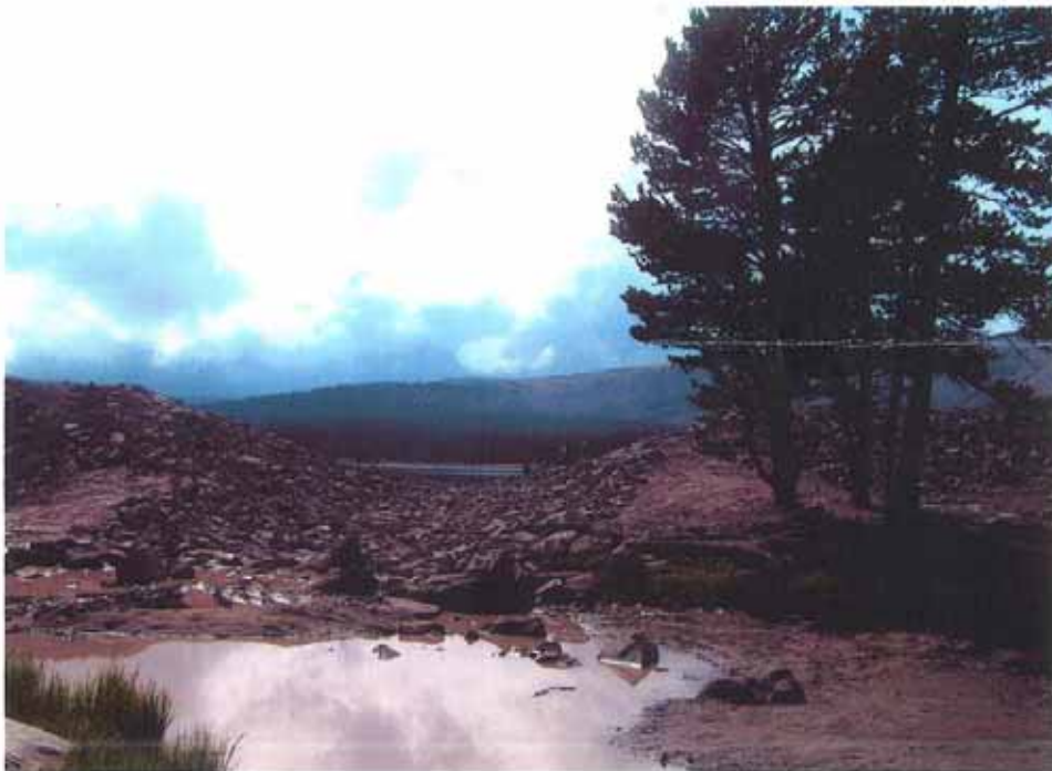
Clement's breach looking upstream.
