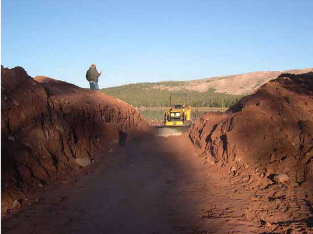
Figure 16 - Starting to widen bottom cut through dam embankment.
