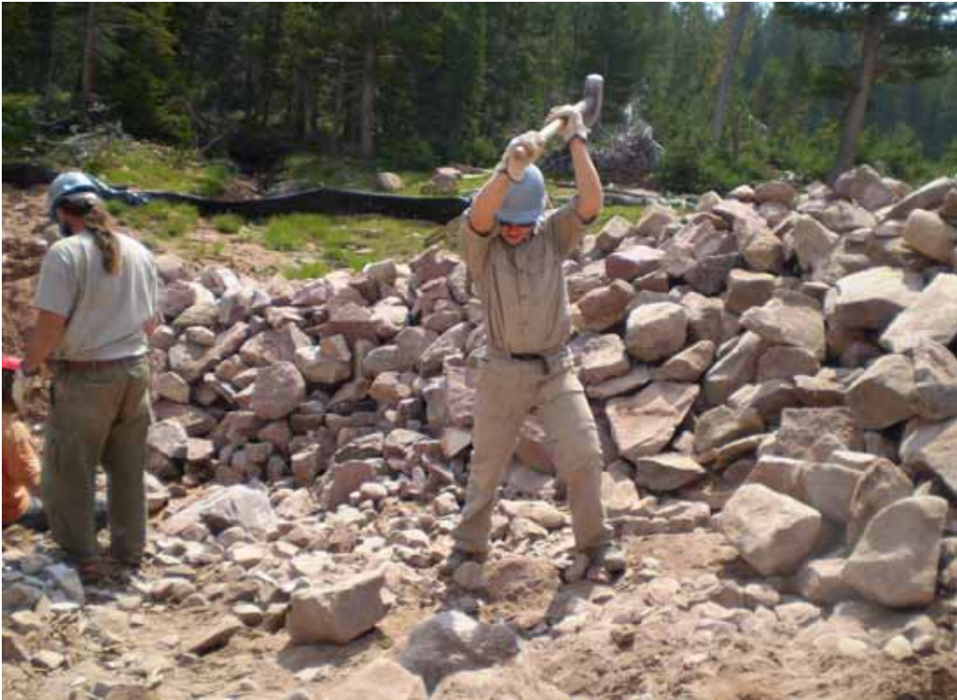
Figure 7 - SCA Crew No. 2 Rock Break Up.
