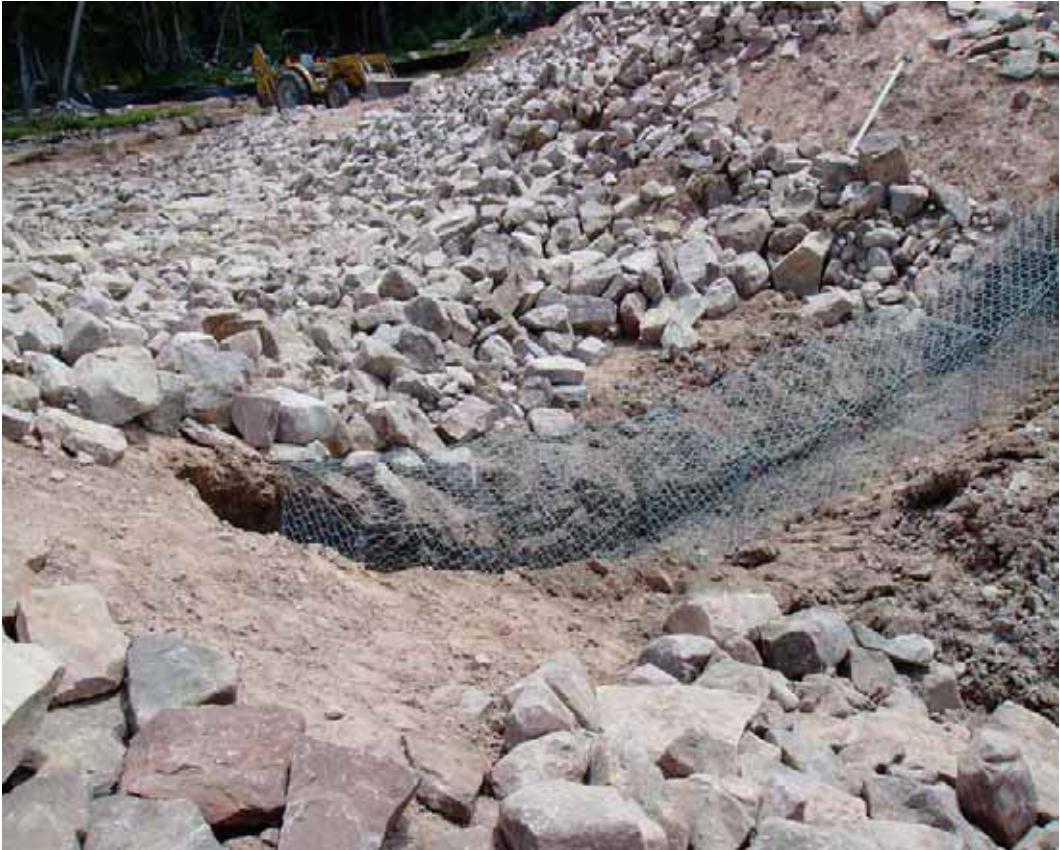
Figure 19 - Installation of the upstream cutoff wall.
