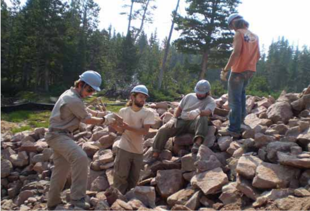
Figure 6 - SCA Crew No. 1 Rock Removal.
