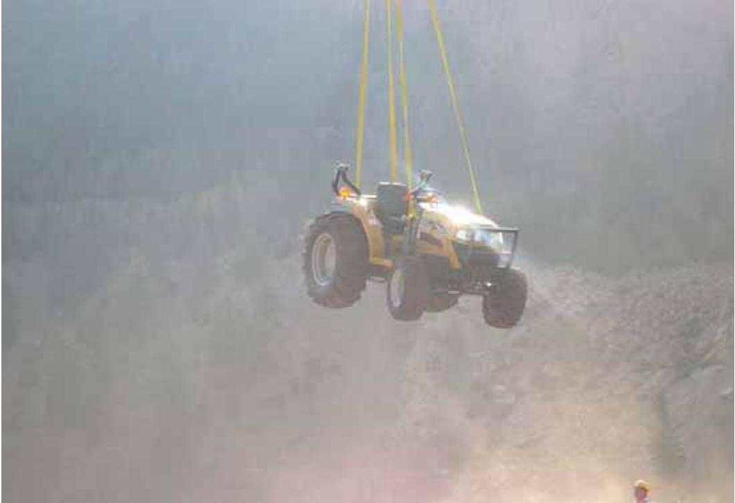
Figure 8 - Challenger tractor being airlifted to worksite from Moon Lake staging site.
