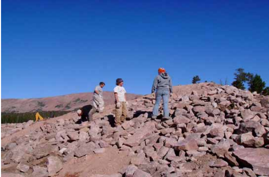
Figure 22 - SCA Crew No. 2 Rip Rap Placement.
