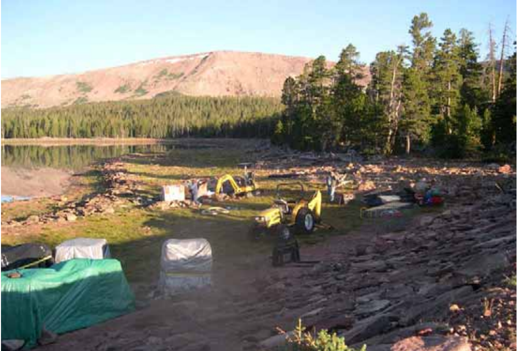
Figure 12 - Equipment and materials layout at upstream face of dam after airlift.
