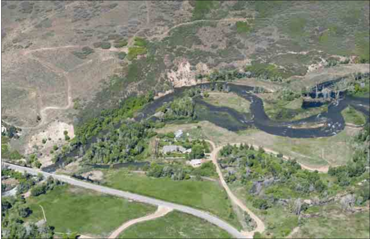
PHOTO 4.2. THE RIVER ROAD (RR) SEDIMENT TRANSPORT MONITORING BRIDGE (BOTTOM LEFT). DIRECTION OF FLOW IS FROM RIGHT TO LEFT. NOTICE THE RESTORED MEANDERS UPSTREAM OF THE ERODING SIDE HILL.
