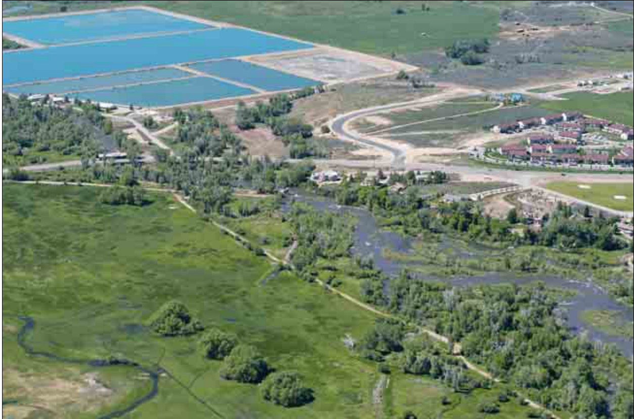
PHOTO 4.3. THE MIDWAY BRIDGE (MID) SEDIMENT TRANSPORT MONITORING BRIDGE (MIDDLE LEFT). DIRECTION OF FLOW IS FROM BOTTOM RIGHT (NEVER-CHANNELIZED PORTION OF THE MIDDLE PROVO RIVER) TO UPPER LEFT (HEBER VALLEY SEWER IMPROVEMENT DISTRICT'S WASTEWATER TREATMENT PONDS).
