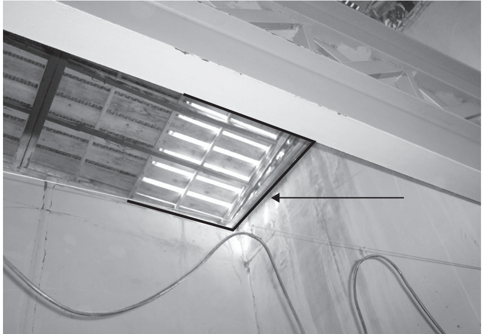
Figure 5: Storage Facility Containing RTGs and a Seed Irradiator with Holes in the Roof
