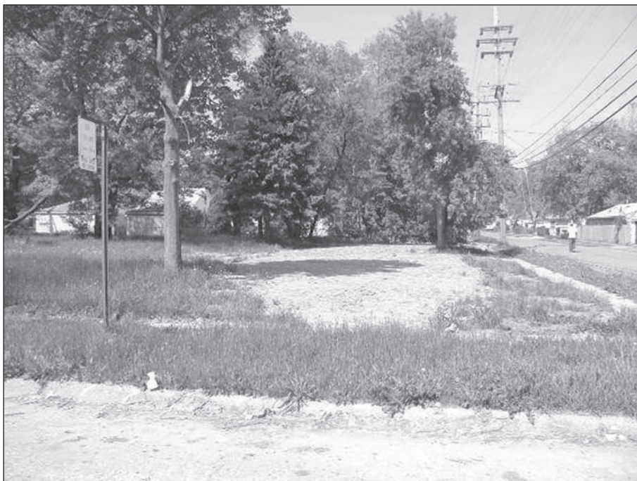
Figure 15: Demolished VA Foreclosed Property
