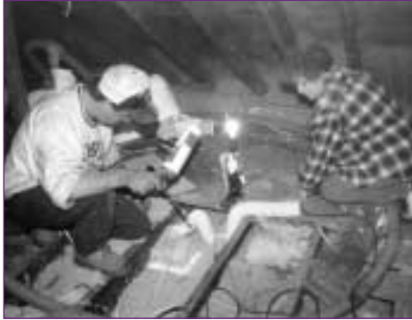
Weatherization crew installs insulation in the attic of a New Jersey home.
