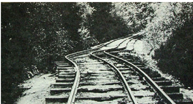
Figure 3-7. Damage to the railroad track between Wrights Station (near the tunnel) and Alma caused by the 1906 earthquake. Both historic settlements and the rail line no longer exist. The gravel road now follows the rail path. The photograph is from an unspecified source reproduced by Iacopi (1969).
