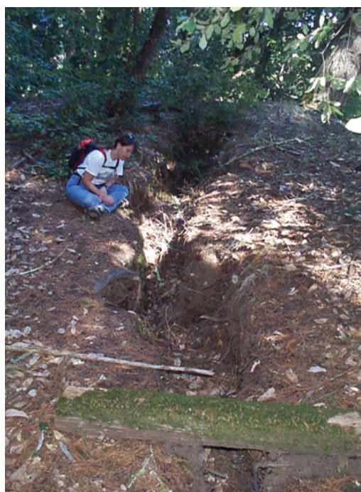
Figure 4-3. One of many fissures that opened along the Big Slide Trail during the 1989 Loma Prieta earthquake.
