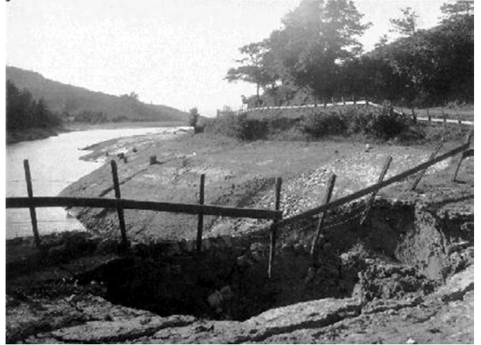
Figure 5-2. Ranch Lake as it appeared shortly after the 1906 San Francisco earthquake. Ground failure in the foreground is the result of slumping of the earthen dam at the south end of the lake. Local lore is that a large quantity of water splashed out of the lake as a result of the earthquake. Note the high water line that existed at the time of the earthquake. Also note the comparative lack of forest in the photo as compared to the modern image below. The main trace of the fault runs along the base of the hill on the left, but the whole lake is within the fault zone. (Photograph from Lawson, 1908.)
