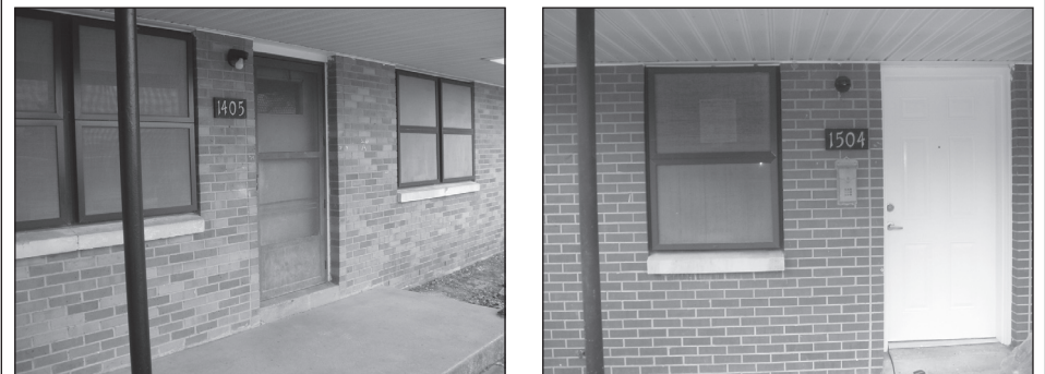
Housing unit with front door scheduled for replacement (left) and housing unit with front door replaced (right).
