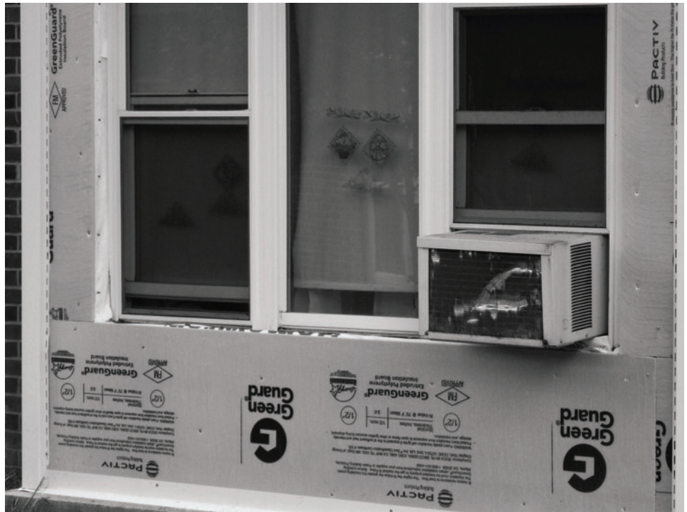
Figure 11: Siding in the process of completion using Rahway Housing Authority's Recovery Act funds
