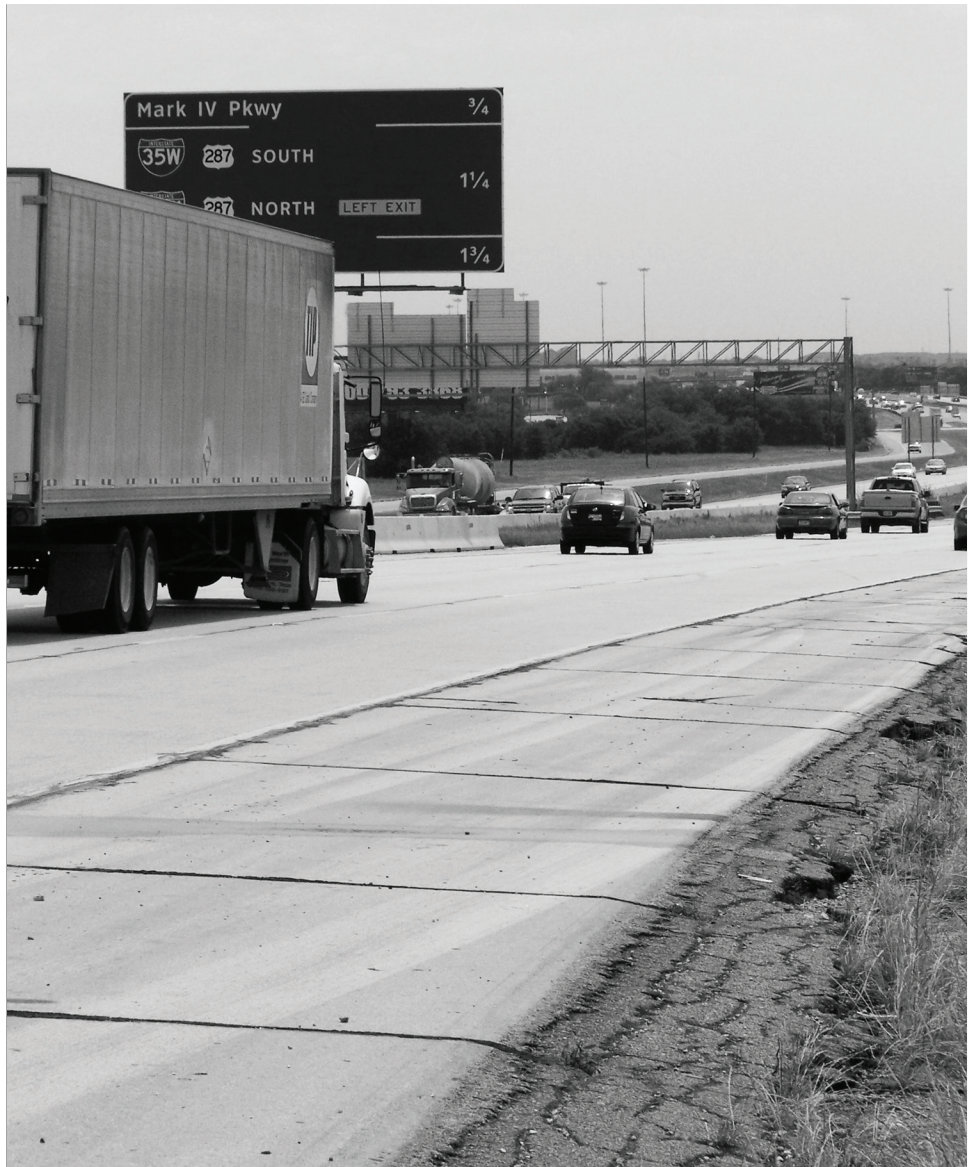
Figure 3: Fort Worth District Roadway Resurfacing
