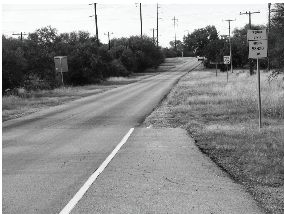
Figure 2: San Antonio District Road-Widening Project
