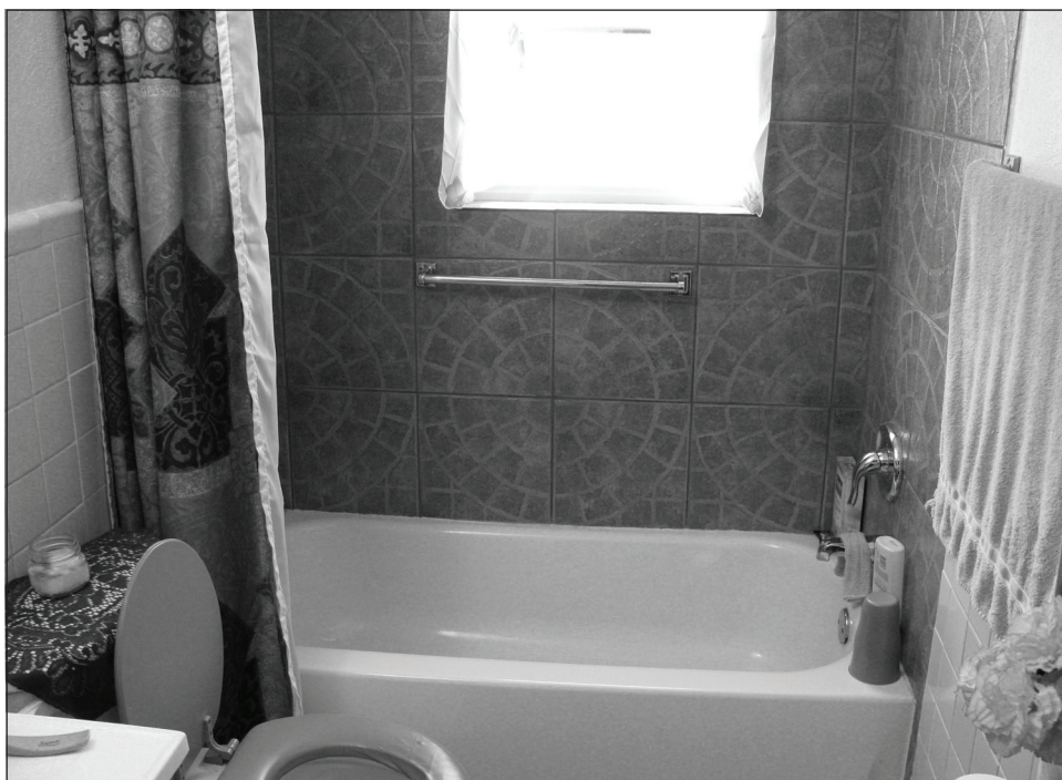
Figure 8: Ferris Housing Authority—Renovated Bathroom with Updated Tile, Bathtub, Toilet, and Sink
