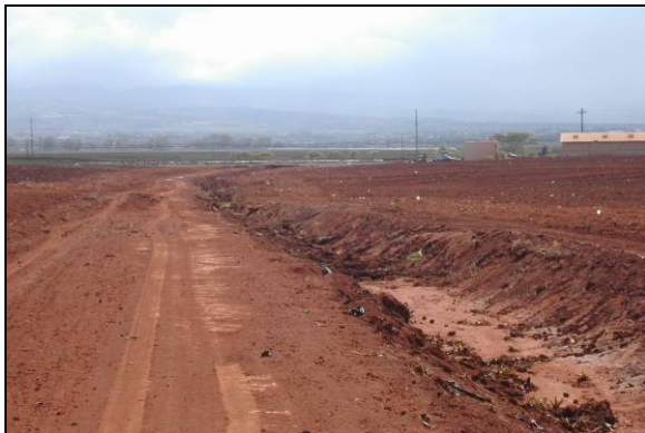
Vetiver site on Oahu before vetiver installation 2005
