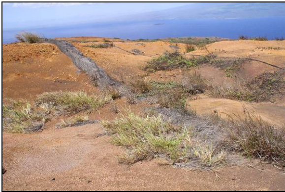
Piligrass wrapped in geotextile fabric were named the bundle or berm method. Native Kamanomano and Piligrass growing along bundles, August 2008
