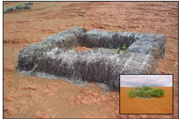
Piligrass hay bales in box configuration installed in 2004 at Moiwi bypass road on Kahoolawe. Photo inset of Aweoweo growing in box October 2005, LZ-3
