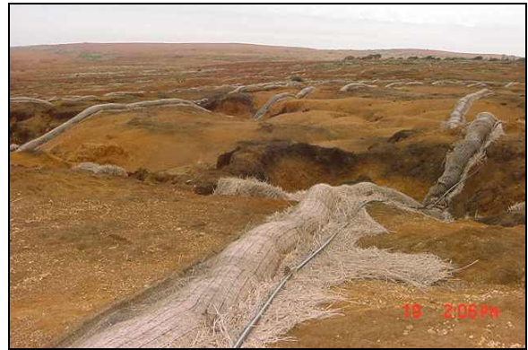
Piligrass bundles installed in 2005 on southeast rim of Lua Makika, Kahoolawe
