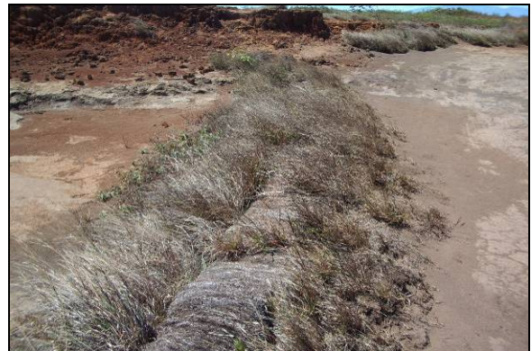
Piligrass bales installed in 2002 continue to trap sediment. Note piligrass growth both up slope and down slope of bales. August 2008
