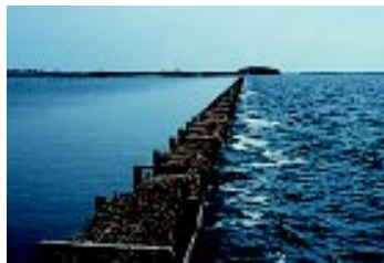
Demonstration projects are small scale and are used to showcase restoration methods. In the photos above and at left, wave-dampening devices protect shorelines and nearby marshes from erosion.
