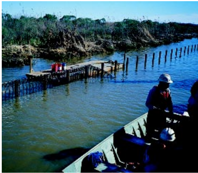
Demonstration projects are small scale and are used to showcase restoration methods. In the photos above and at left, wave-dampening devices protect shorelines and nearby marshes from erosion.
