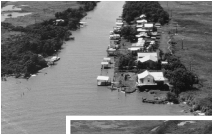
The photo above shows the junction of Boston Canal and Vermilion Bay before project construction. Water was displacing marsh ground and encroaching on local structures.
