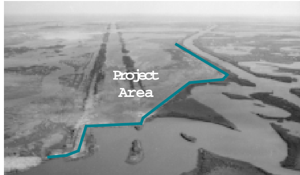
The West Belle Pass project area is situated behind the blue lines above. As dredged material is pumped into the project area, dry land eventually rises out of the open water and becomes marsh. (ACOE photo)
