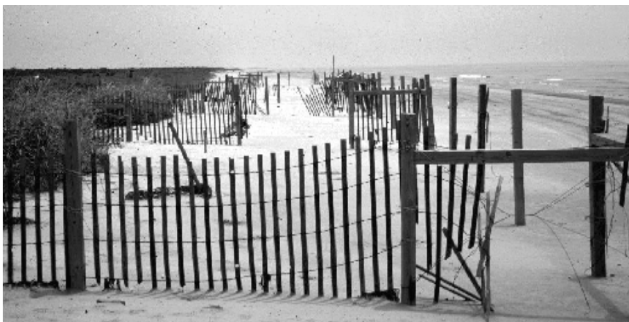
In some projects, success is hard won. The photo above reveals some of the damage suffered by sediment-trapping fences at Timbalier Island from storms in the Gulf of Mexico. (NRCS photo)
