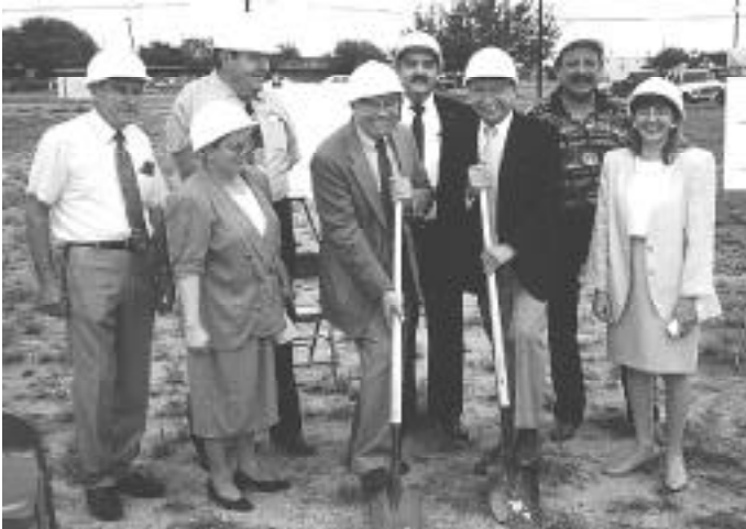
August 15, 1995 — Chairman Norman E. D'Amours (center right) helps break ground for LaJoya Teachers FCU, TX, new headquarters. The Chairman visited 6 of the 44 limited-income credit unions in Texas during a two-day visit in mid-August.
